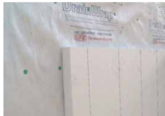
Figure V: DuPont™ Tyvek® DrainWrap® Under Foam Sheathing
