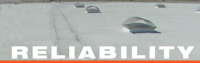
In 1996 and 2003, the National Roofing Foundation commissioned Dr. Rene Dupuis of Structural Research Inc. to conduct an extensive study¹ of SPF roofing systems. The study included over 300 SPF roofs in six different climate zones around the United States. A conclusion from this completely independent study was that SPF roofs have an effective service life of more than 30 years.
