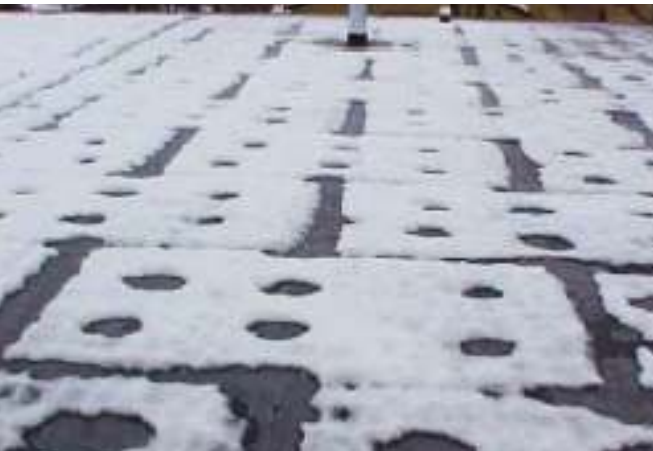
[ Snow on single ply roof melting where thermal bridging occurs. ]
