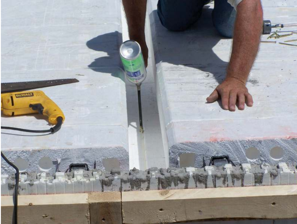
Figure 4.3 – Sealing seam between AmDeck™ blocks
