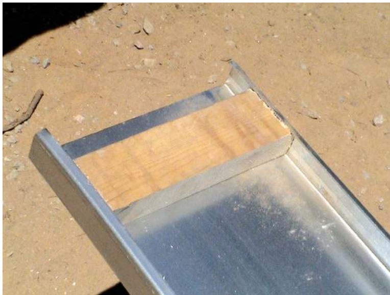
Figure 7.17 - Inserting a wood block in the steel joists
