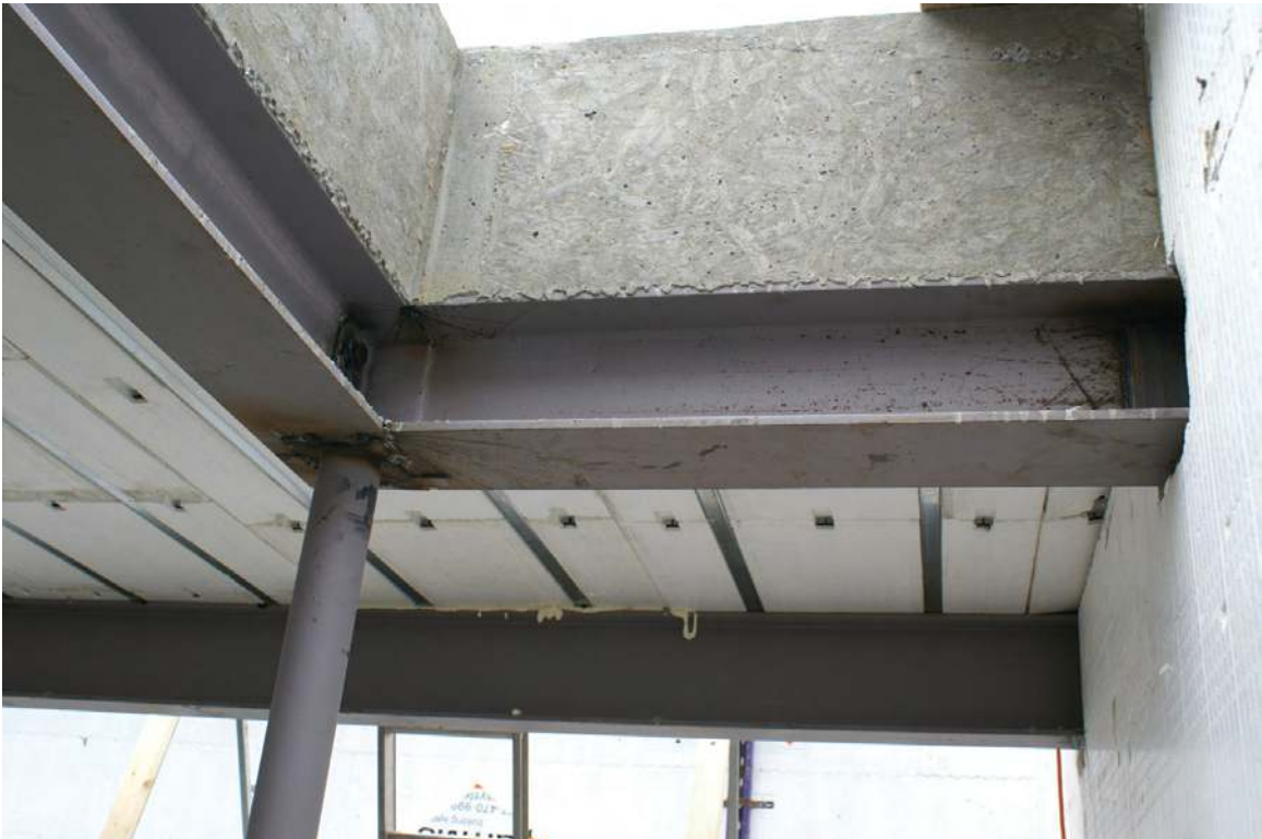
Figure 6.14 – Large sized opening in AmDeck™ supported by steel perimeter beam and column.
