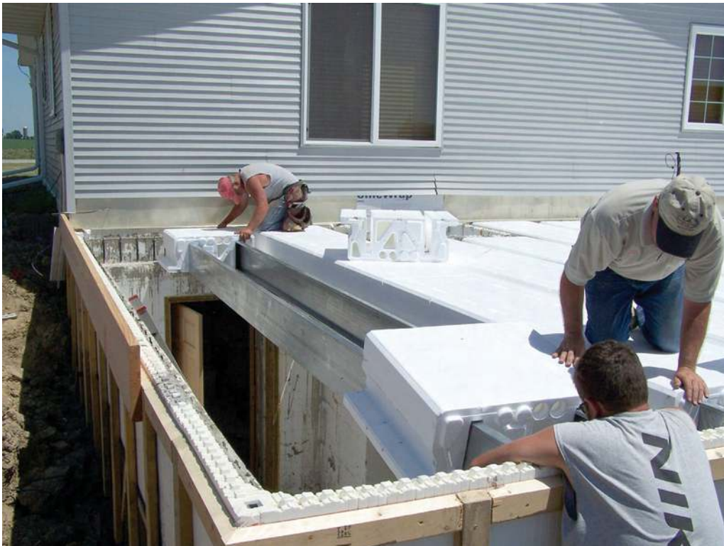
Figure 7.7 - Installing the AmDeck™ Blocks at each end of steel joist pair
