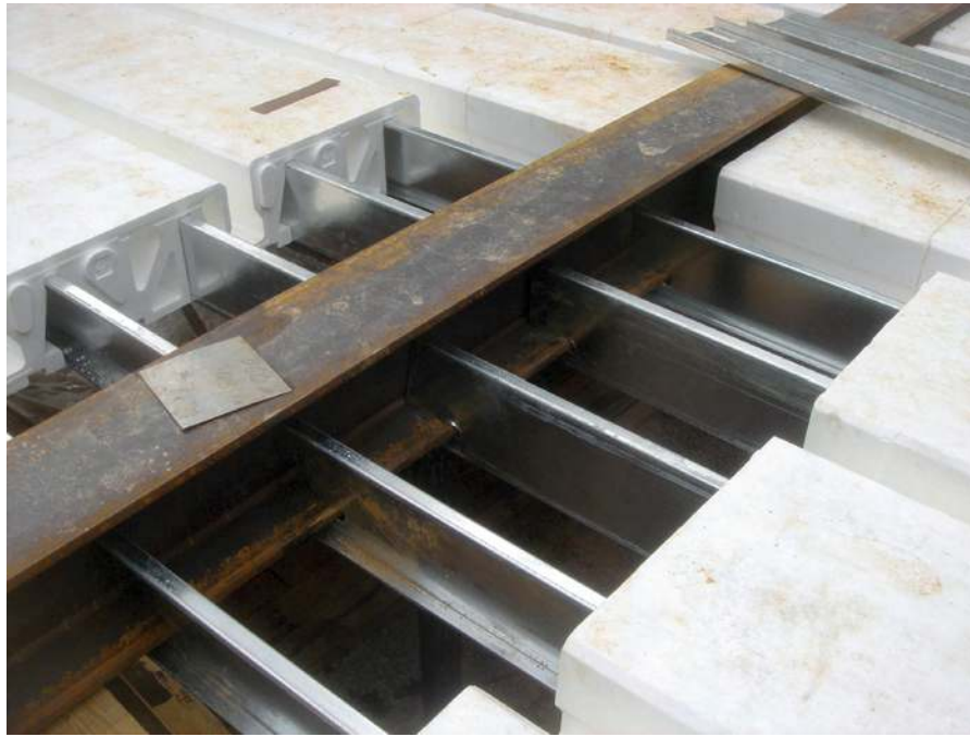
Figure 7.26 – Connection between steel joists and steel beam
