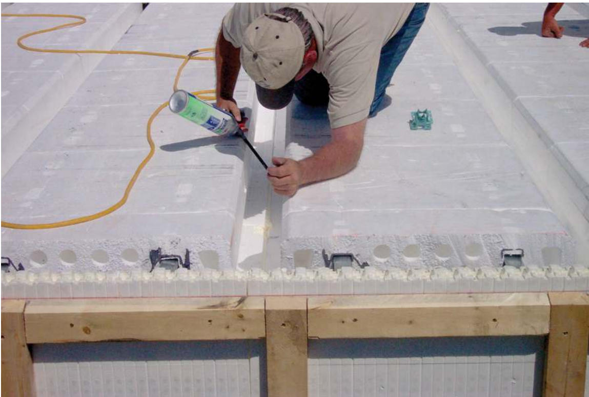
Figure 7.15 – Sealing gaps between AmDeck™ forms
