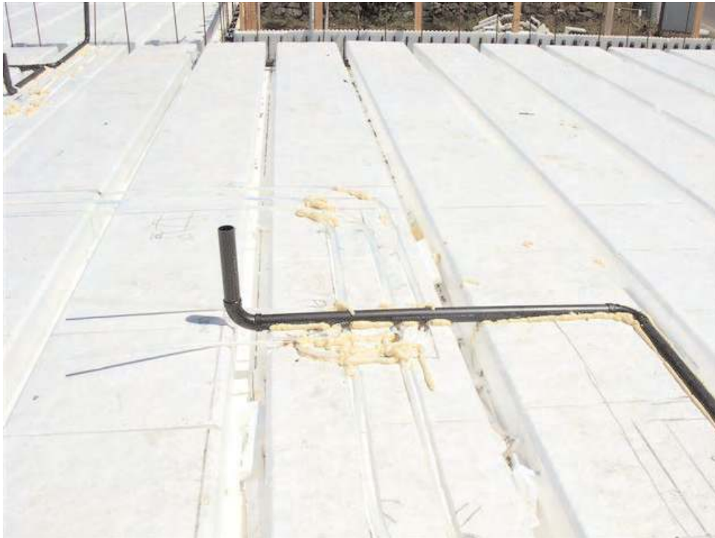
Figure 7.18 – Pipe placed in the AmDeck™ top slab region.
