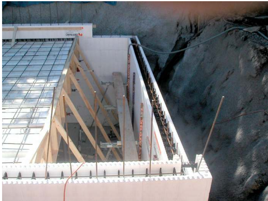
Figure 7.25 – Bracing the formwork for concrete beam
