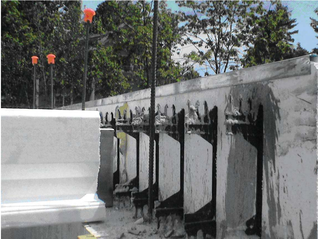
Figure 7.20 - Amvic ICF cut halfway
