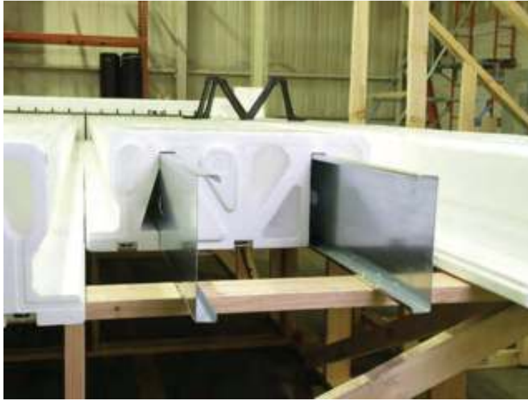
Figure 7.6 – Steel joists placed correctly with C-channels facing each other
