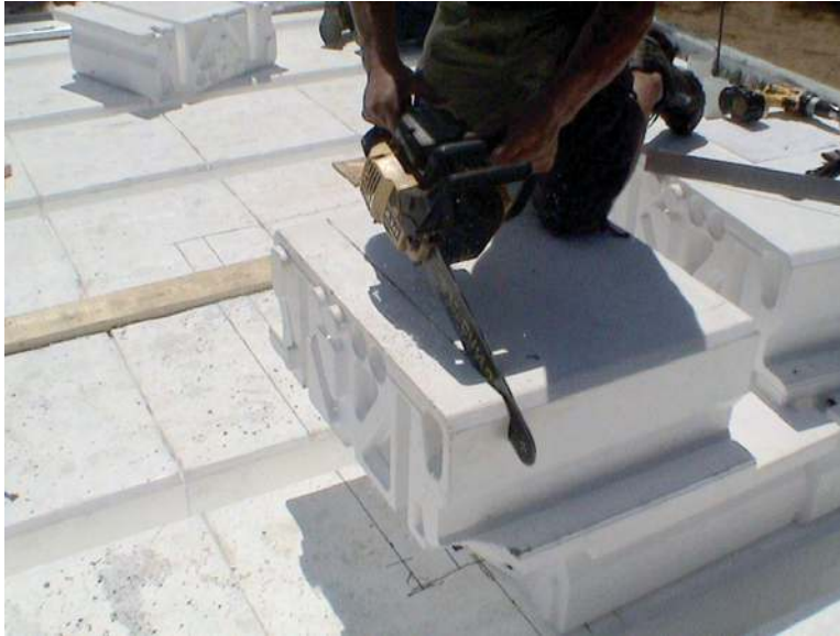
Figure 7.10 - Cutting the final block in the row
