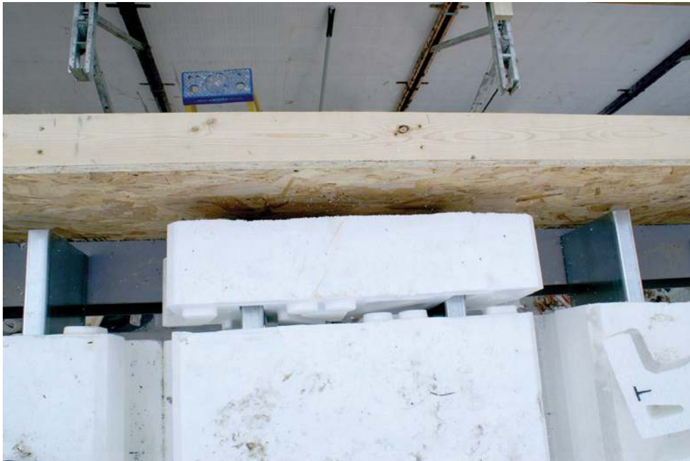
Figure 7.11 – Placement of AmDeck™ block cut transversally
