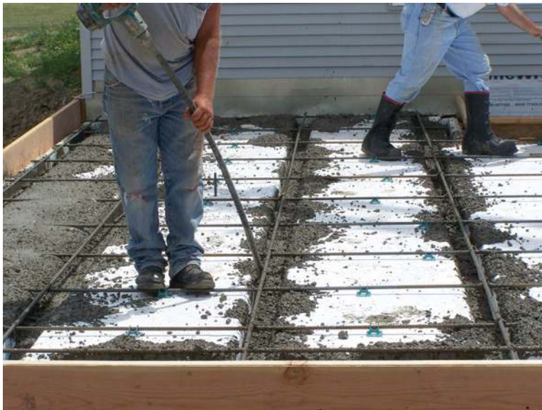
Figure 4.5 – Consolidating concrete on AmDeck™ using a mechanical vibrator
