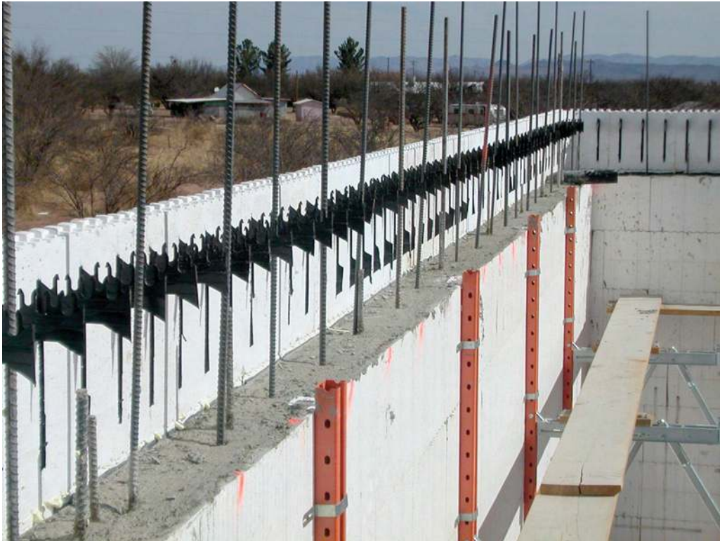
Figure 7.21 - Another view of Amvic ICF cut halfway
