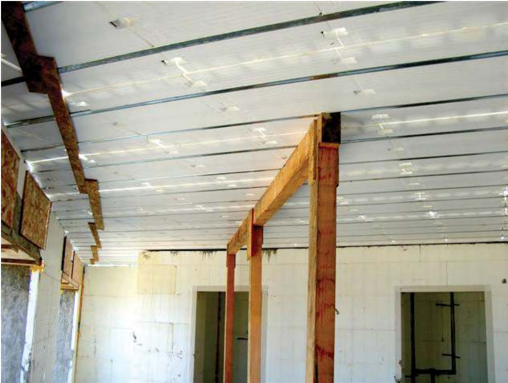
Figure 7.28 – Extra bracing for AmDeck™
