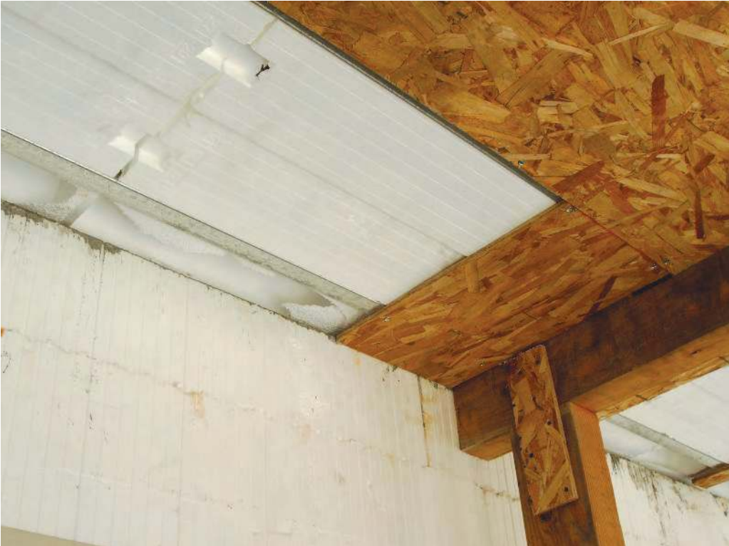
Figure 7.14 – Longititudinally cut AmDeck™ block, supported by OSB board
