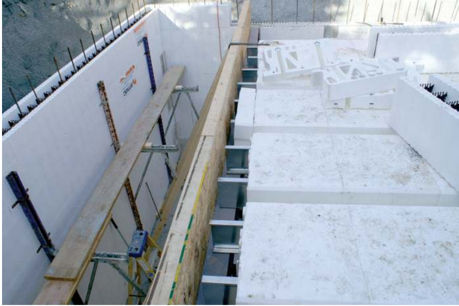
Figure 7.24 – Formwork for concrete beam construction
