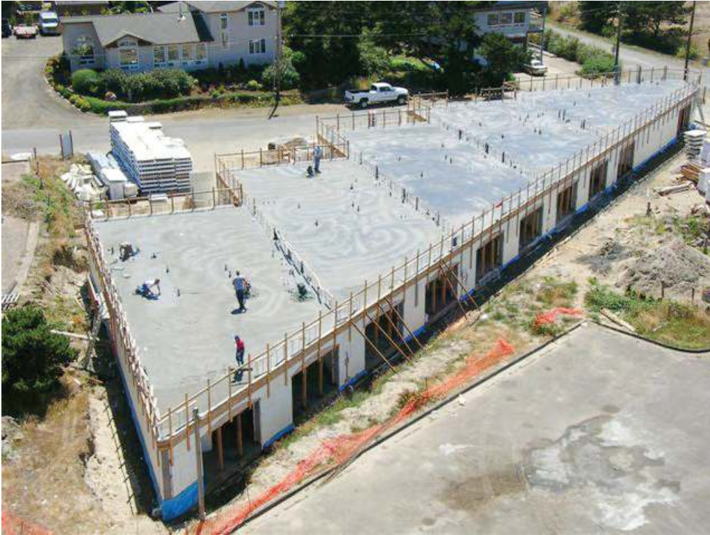
Figure 7.23 - Using guardrail uprights and horizontals to brace perimeter of wall
