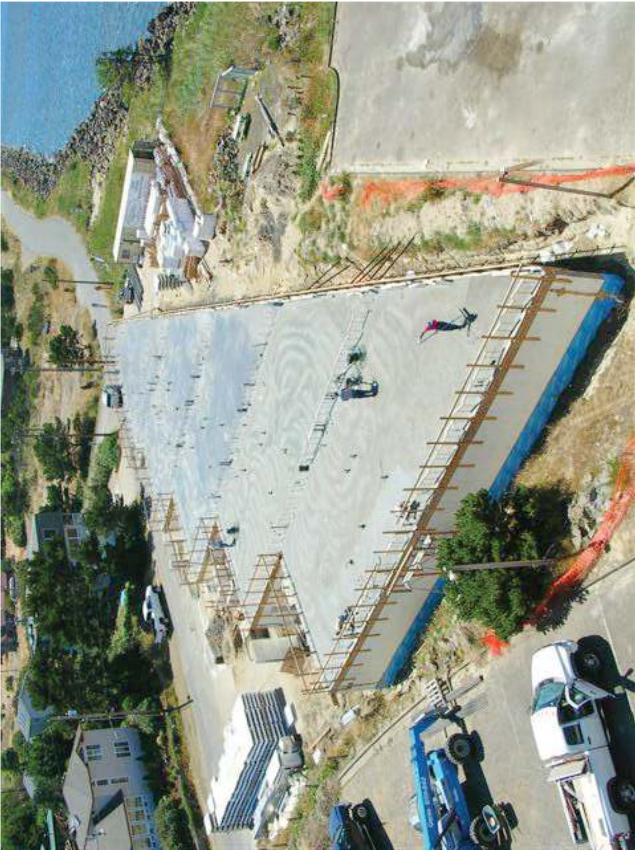
Figure 8.8 – Stage 2: Final Finishing of Concrete on AmDeck™
