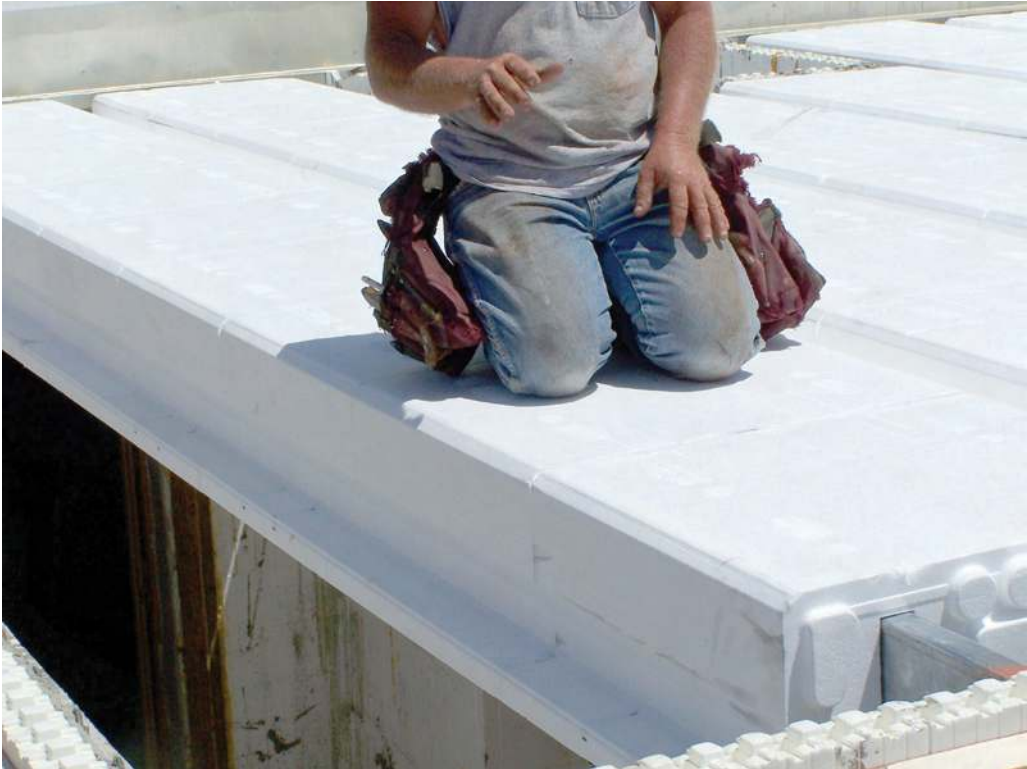
Figure 7.12 – A completed AmDeck™ row
