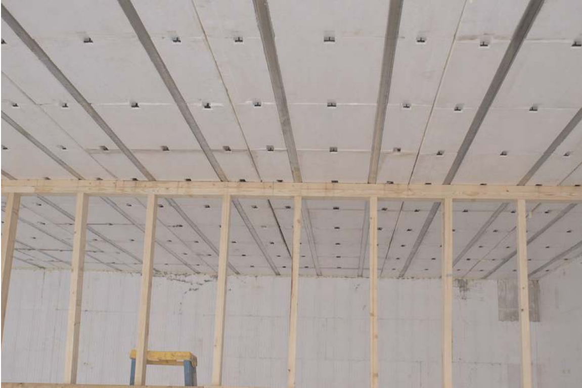
Figure 4.2 – Shoring beneath AmDeck™ floor
