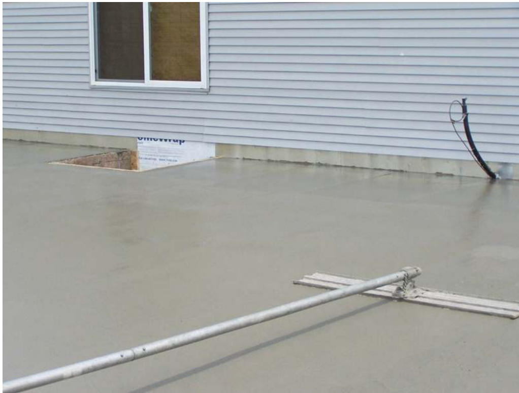
Figure 4.6 – Finishing concrete surface on AmDeck™
