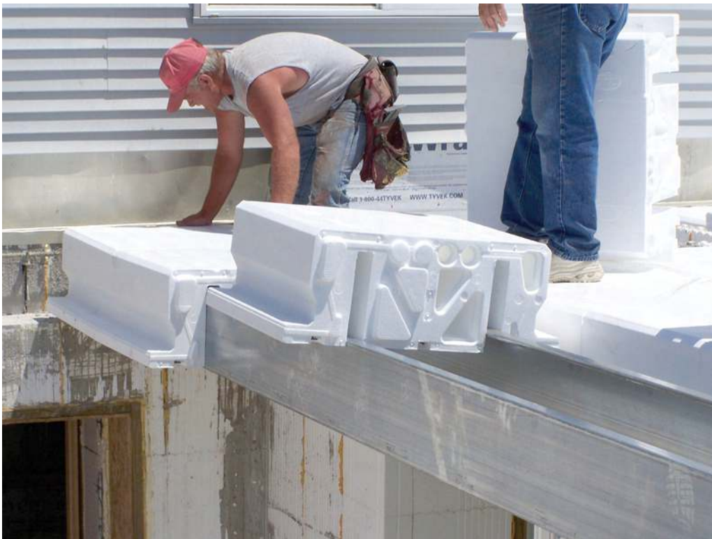
Figure 7.8 - Installing AmDeck™ blocks from one end to the other
