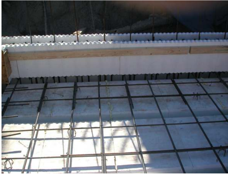
Figure 4.4 – Transverse and longitudinal steel on AmDeck™ for top slab
