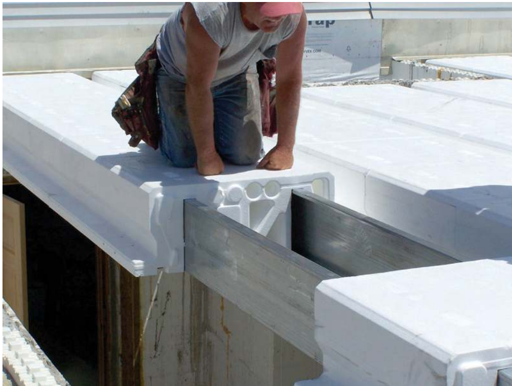
Figure 4.1 – Laying out forms
