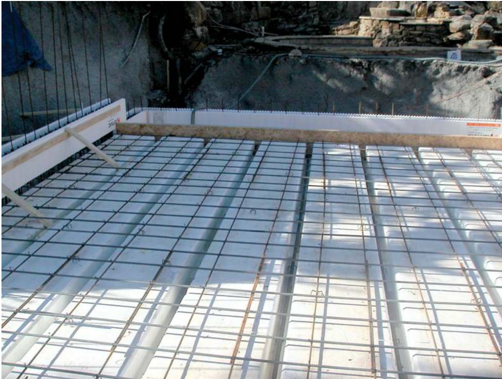
Figure 7.19 - Transverse and Longitudinal Steel
