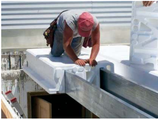
Stacking the AmDeck® Floor & Roof System.
