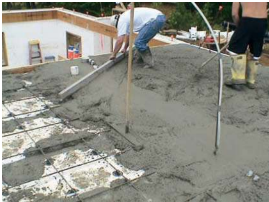
Smoothing concrete to create a flat surface.
