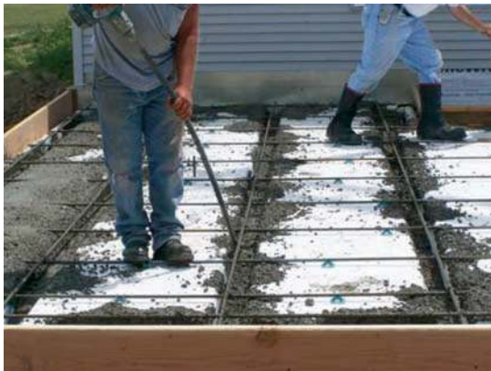
Pouring concrete onto the assembled forms.
