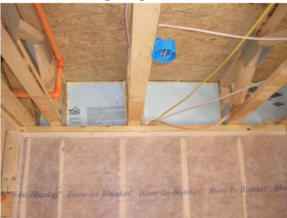
Figure 4. The I-joist is continuous along the shared wall and serves as a natural air barrier between the garage and the house. (Image courtesy of CARB)
