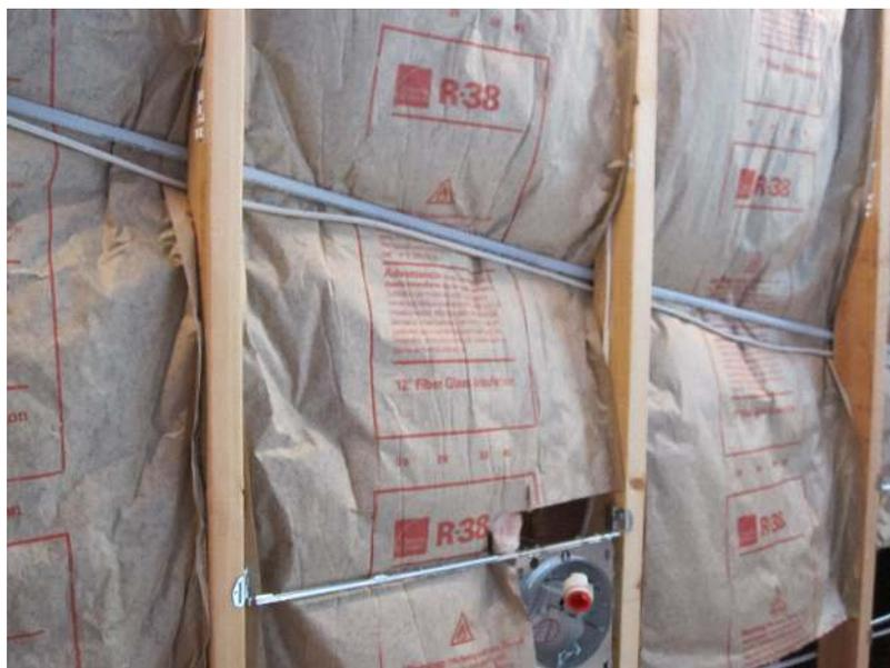
**Figure 2** - This faced fiberglass batt insulation was incorrectly installed; it should be cut to fit around wiring and obstructions so that it can completely fill the wall cavity without compressions and voids. [i](#)
