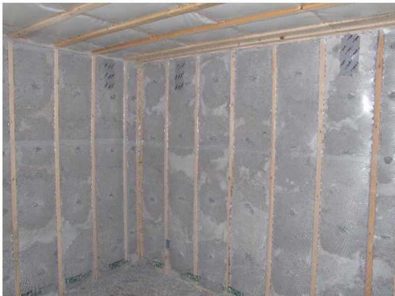
**Figure 4** - Blown cellulose insulation completely fills the netted wall and ceiling cavities and flows easily around wiring and other obstructions to provide a uniform insulating layer without gaps or voids. ⓘ
