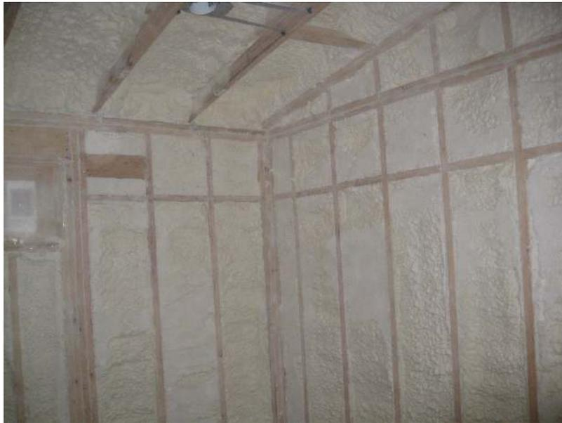
**Figure 5** - Spray foam insulation is installed in open wall cavities to air seal and insulate.
