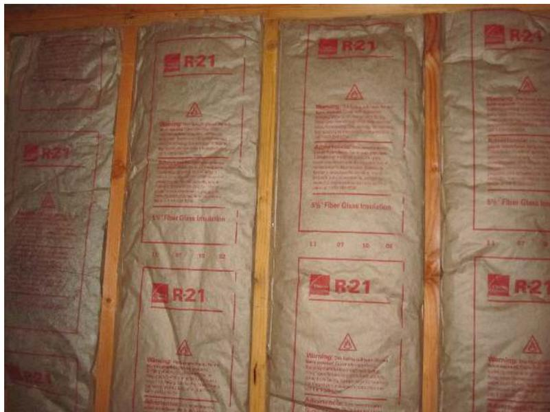
**Figure 6** - Faced fiberglass batt insulation can be stapled to the stud faces or slightly inset, but avoid compressing the batts and slit the insulation to fit around wiring and other obstructions.
