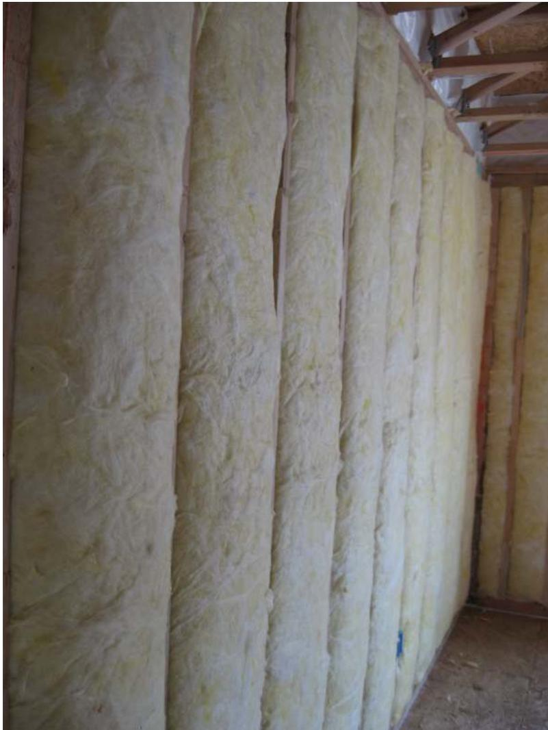
**Figure 1** - Unfaced fiberglass batt insulation is installed to completely fill the wall cavities and is sliced to fit around wiring, piping, and other obstructions in the wall cavities. [i](#)
