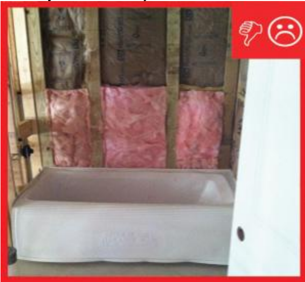
Display Image: JM_behind-tub-missing-air-barrier-2_wrong_TE.jpg Courtesy Of: Jim Mackovyak
