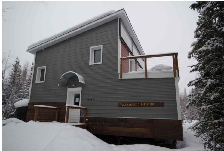
Figure 2. Tamarack house. This house has 5.5 inches (14 cm) of fiberglass batt in the stud space and 8 inches (20cm) of rigid polystyrene foam on the outside of the sheathing.
