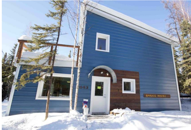
Figure 9. Spruce house. This house has 5.5 inches (14 cm) of fiberglass batt in the stud space and 12 inches (30.5 cm) of dense pack cellulose on the outside of the sheathing.
