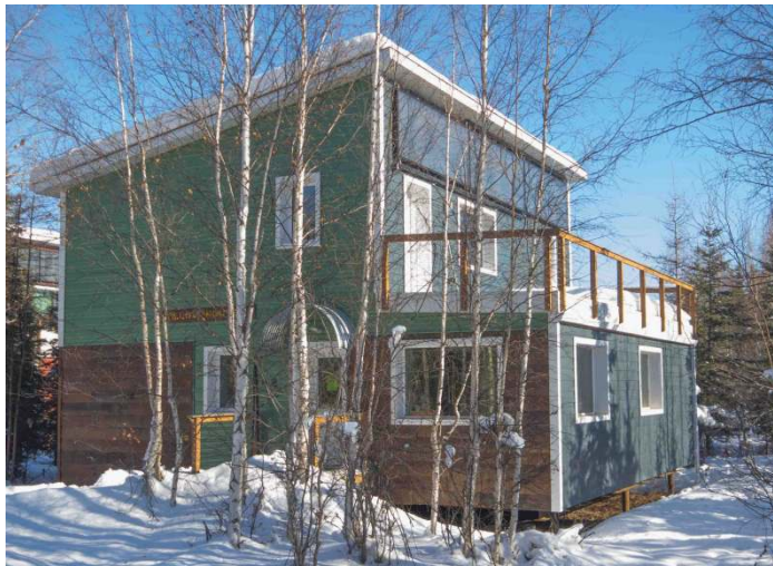
Figure 7. Willow house. This house has 5.5 inches (14 cm) of fiberglass batt in the stud space and 8 inches (20cm) of rigid polystyrene foam on the outside of the sheathing.
