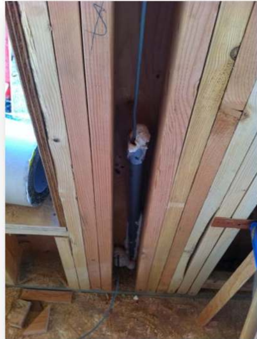
Figure 6. Temperature (black) and humidity (white) sensors were installed on the interior side of air barrier system (taped sheathing, left photo) and on exterior side of air barrier system (right photo).
