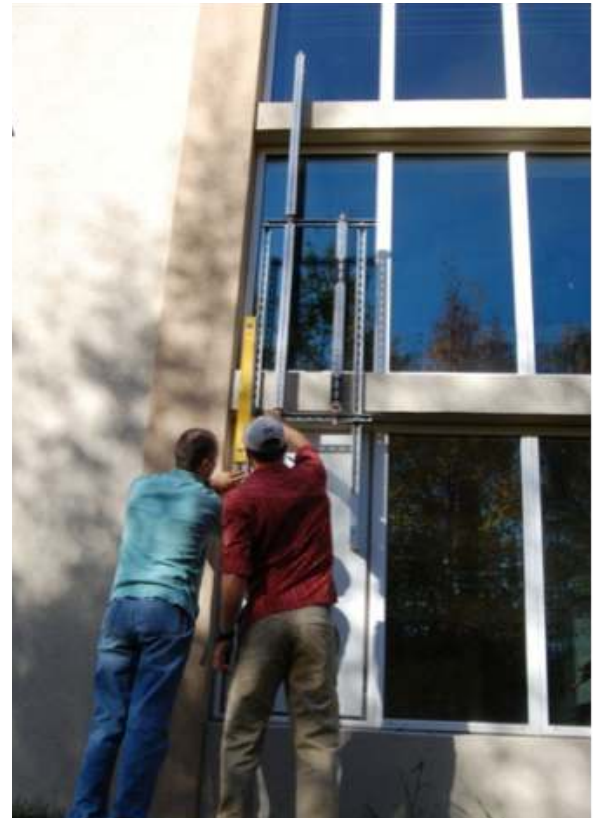
Figure 6. Fins being attached to the building. The freezer section is 8 feet long; the fins were not the limiting heat transfer mechanism of the design and could probably be much smaller.
