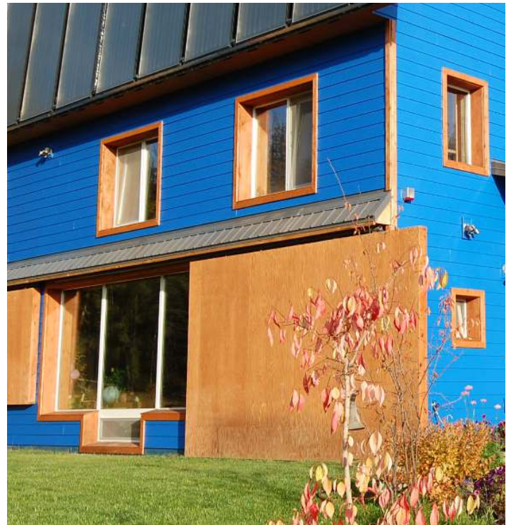
Figure 2. Exterior shutters were one of eight types of window insulation tested in the original study for energy performance, condensation resistance, and other criteria.
