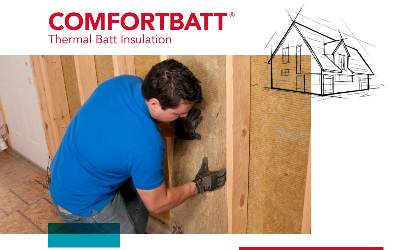
ROCKWOOL COMFORTBATT® is a semi-rigid stone wool batt insulation for exterior wood and steel stud applications in both new construction and renovations.
