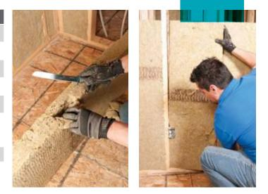
ROCKWOOL cuts quickly and accurately with a serrated knife, such as a bread knife, so you can easily achieve optimal fit around pipes, electrical boxes, wiring, ductwork and between studs and joists that are less than a standard width.
