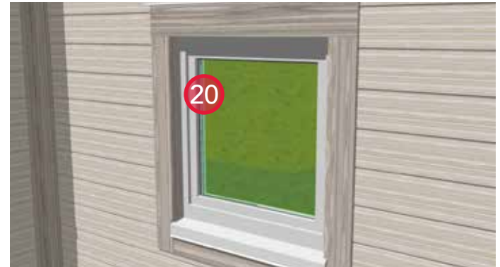
20. Install cladding.
