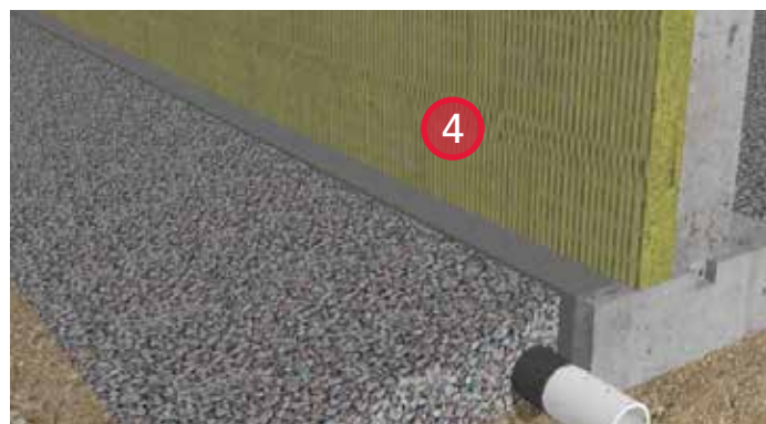
4. Install ROCKWOOL rigid board insulation against foundation wall. Spot adhere the insulation to prevent puncture of the waterproofing membrane.
