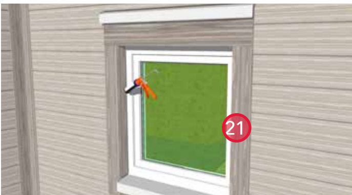
21. Install sealant around the perimeter of the window between the trim boards and the window frame (top and sides).
