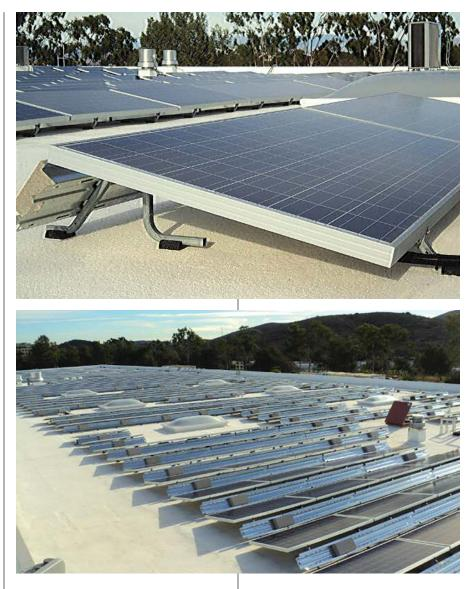
coatings and granules will help protect the roof during this time, as well as during scheduled maintenance. Because a roof surface below PV panels will likely not dry as fast as non-covered portions, coatings that stand up better to standing water and biological growth should be selected.
