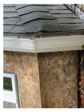
intersection leaks. A kick-out diverter would reduce potential for water intrusion at this leak-prone location. A logical and economical solution to reducing water intrusion and reduce liability claims is to consider a seamless pre-molded polymer-based product.
