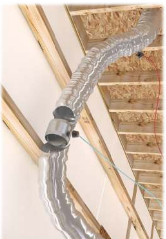
Motorized damper and temp. sensor
