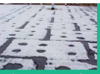
Snow on single ply roof melting where thermal bridging occurs.
