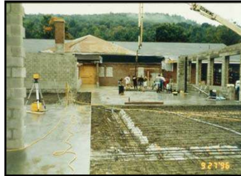
Sand layer taking on water from rainfall
