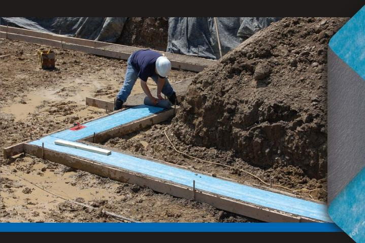
Resists capillary rise of moisture in foundations.
