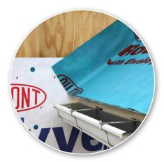
**STEP 1** Apply drip edge and roof underlayment over roof deck. Continue lapping up the sidewall and over the water-resistive barrier (in this case housewrap) a minimum of 6 inches.
