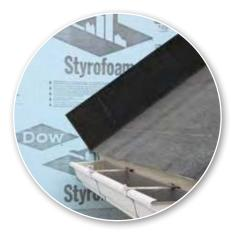
**STEP 1** Apply drip edge and roof underlayment over roof deck and continue lapping up the sidewall and over the water-resistive barrier (in this case rigid foam insulation) a minimum of 7 inches.
