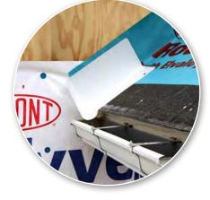
**STEP 2** Install shingle starter strip at roof eave in accordance with roofing manufacturer's instructions.
