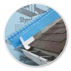
**STEP 6** Apply construction tape over the self-adhered flashing.
