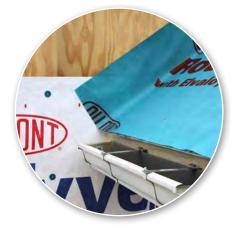
**STEP 1** Apply drip edge and roof underlayment over roof deck. Continue lapping up the sidewall and over the water-resistive barrier (in this case housewrap) a minimum of 6 inches.
