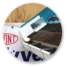
**STEP 3** Place first shingle and next section of sidewall flashing over the up-slope edge of diverter, lapping a minimum of 4 inches over diverter. (Sidewall flashing height requirement should be determined by design professional and local building codes.)
