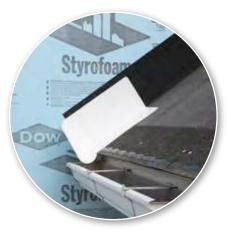
**STEP 2** Install shingle starter strip at roof eave in accordance with roofing manufacturer's instructions.
