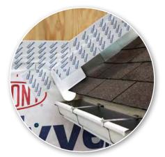
**STEP 5** Apply self-adhesive flashing over top of wall flashing, diverter, and housewrap.
