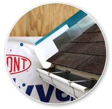
**STEP 4** Install remaining sidewall flashing, appropriate counter flashing, and shingles in accordance with manufacturer's instructions.
