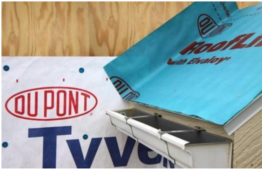
Step 2. Install shingle starter strip then kick-out diverter; attach to roof deck but not sidewall:
