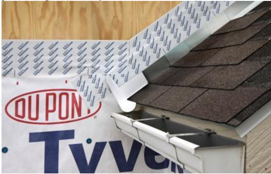
Step 5. Apply self-adhesive flashing over top edge of the wall flashing, diverter, and housewrap:
