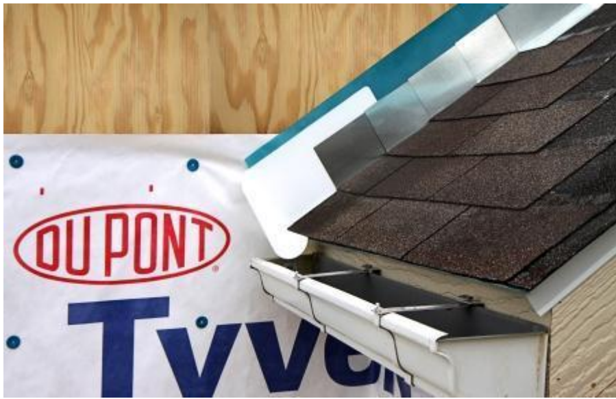
Step 5. Apply self-adhesive flashing over top edge of the wall flashing, diverter, and housewrap:
