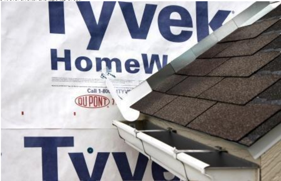
Step 6. Install the housewrap. Cut housewrap to fit over diverter and tape top of cut:
