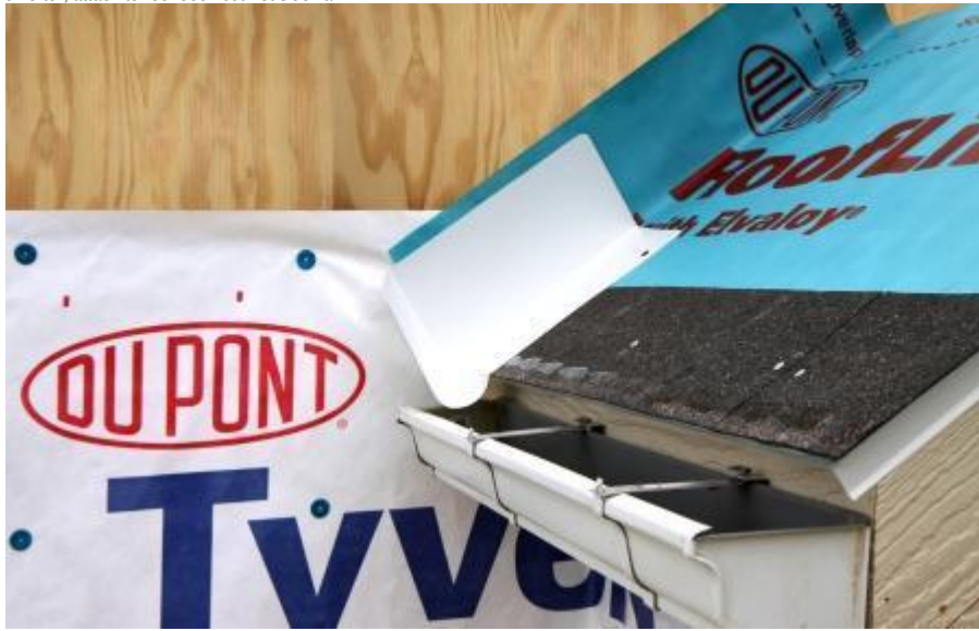
Step 3. Place first shingle and next section of sidewall flashing over upper edge of diverter:
