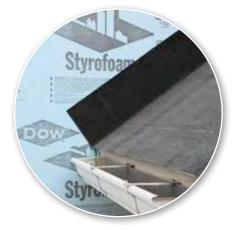
**STEP 1** Apply drip edge and roof underlayment over roof deck and continue lapping up the sidewall and over the water-resistive barrier (in this case rigid foam insulation) a minimum of 7 inches.
