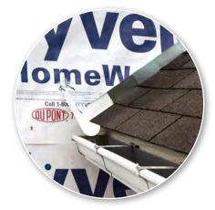
**STEP 6** Install house wrap; cut the house wrap to fit over the self-adhesive flashing and sidewall flashing.
