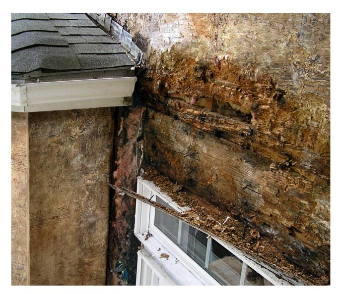
Roof-to-Wall Damage Photo - (Kick-Out Diverter Flashing Not Installed)
