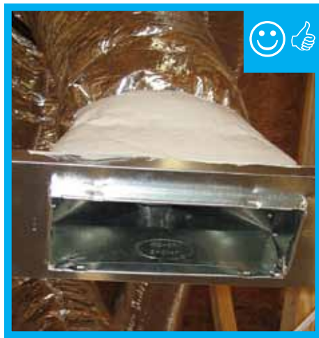
Boot has been covered with insulation and sealed with mastic.
