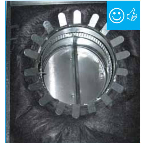
Mechanical damper installed.
