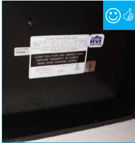
Fan CFM rating is higher than the requirement increasing the likelihood that it will meet the performance level once installed.
