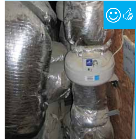
In line exhaust ventilation installed.
