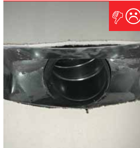
A. Boot to drywall connection not sealed.
