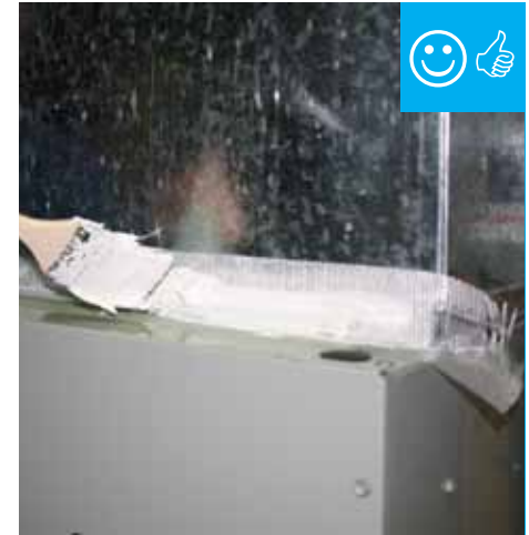
Seams are being properly sealed with mastic and mesh tape.
