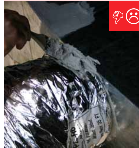
B. No mechanical damper installed.
