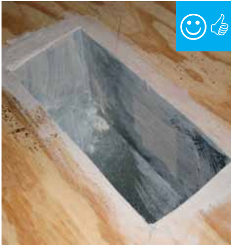
Boot to floor connection sealed.
