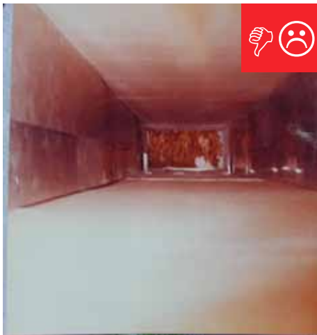
D. Cavity was not air sealed.
