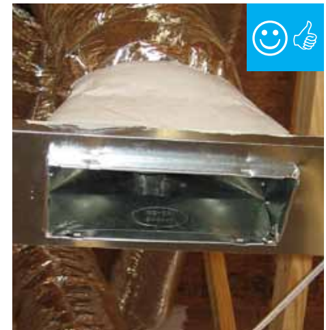
Boot has been covered with insulation and sealed with mastic.
