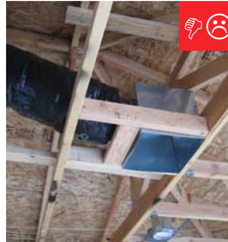
B. Return box has not been sealed.
