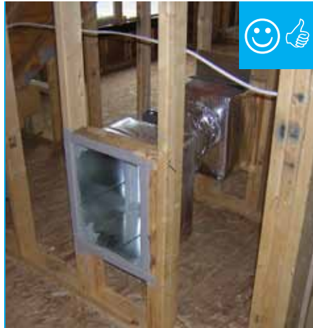
A. Grill and duct size based on calculated requirements for net free area.
