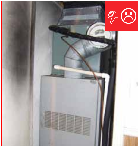
A. Naturally drafted heater installed. Requires combustion safety testing.
