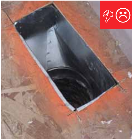
A. Boot to floor connection not sealed.
