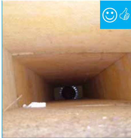
Cavity used for duct has been lined with rigid insulation and is ready to be air sealed.
