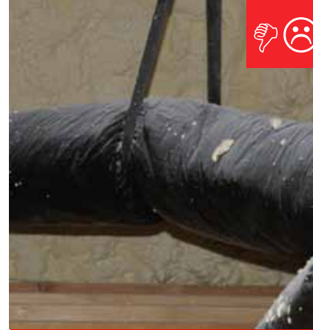
B. Duct is insulated but strapping is compressing the insulation therefore reducing the R-value.
