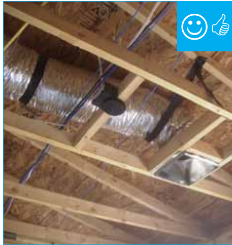
Duct is run straight and supported properly.
