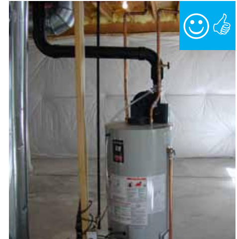
Power vented water heater installed.
