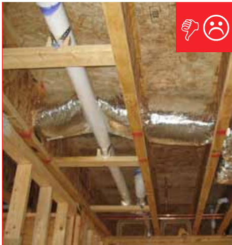
A. Duct is compressed.
