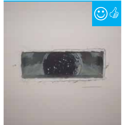
Boot to drywall connection sealed.
