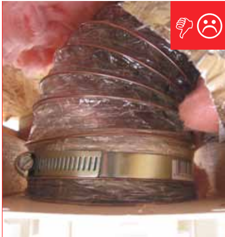
A. Connection in place but not sealed.
