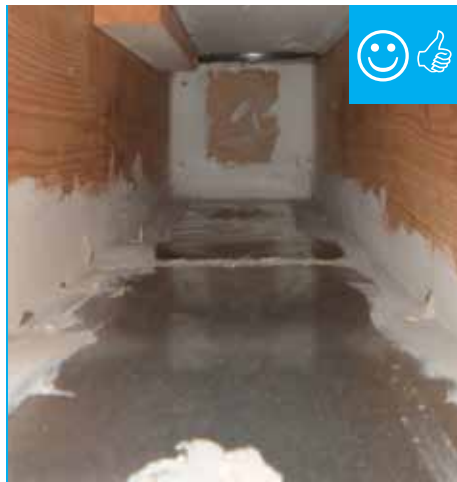
Cavity has been air sealed with mastic.
