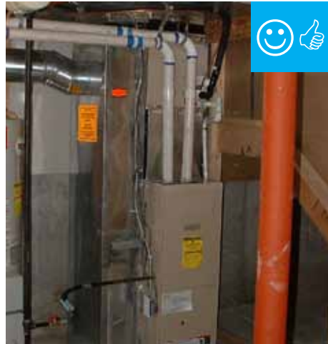
Direct vent appliance installed.
