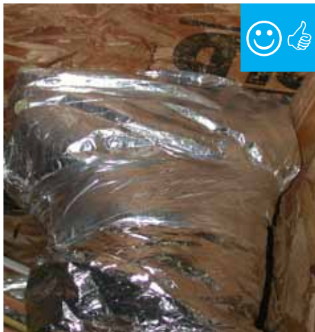
Duct insulation is installed over boot.
