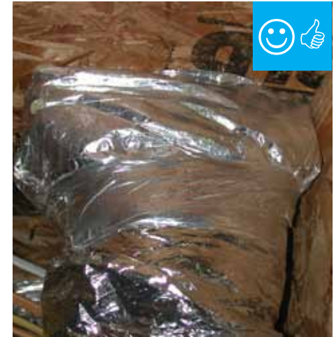
Duct insulation is installed over boot.
