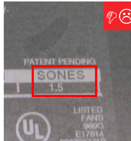
C. Sone rating is greater than 1 on a continuous exhaust fan.
