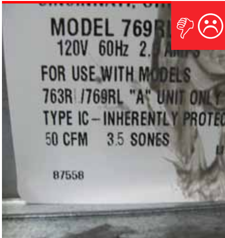
A./B. CFM rating may not meet the performance specification once installed.
