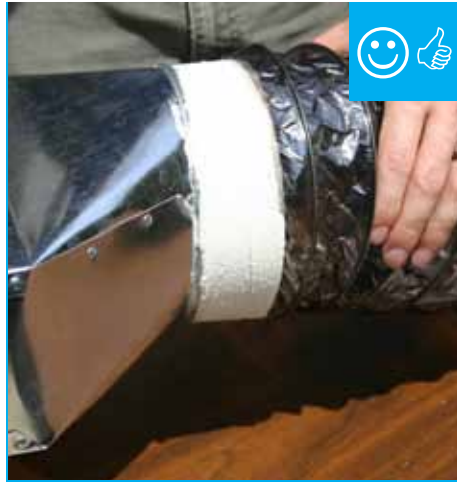
Mechanically fastened and sealed.
