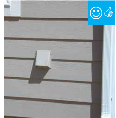
Ventilation inlet is appropriately located above grade.
