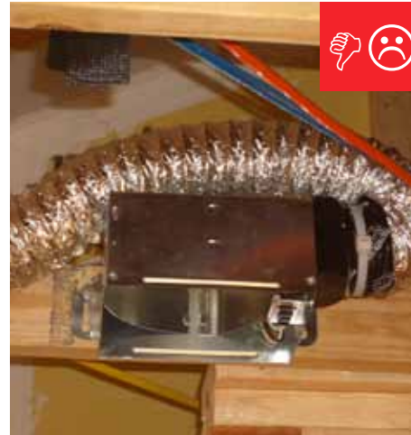
B. Exhaust fan installed but in wrong direction causing excessive bend and duct is uninsulated.
