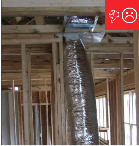
A. Duct is compressed.
