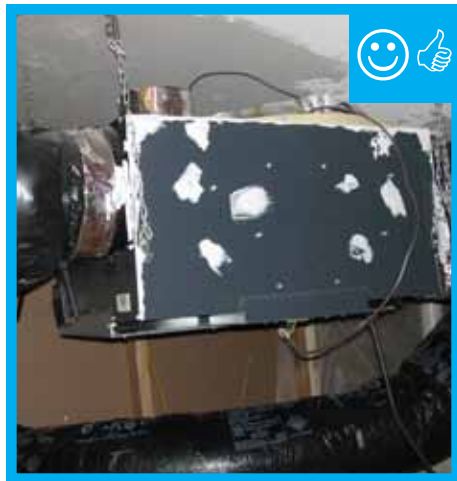
Properly installed ERV/HRV.
