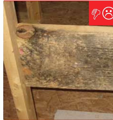
Building materials with visible signs of mold have been used.
