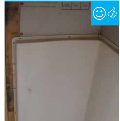
Moisture resistant backing material has been used above the tub enclosure.
