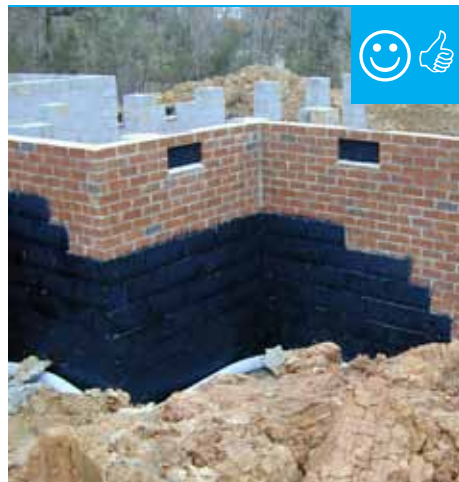
The below-grade concrete walls have damp-proof coating.
