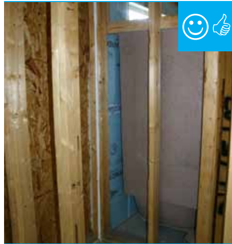
Foam board taped at seams installed behind shower enclosure.
