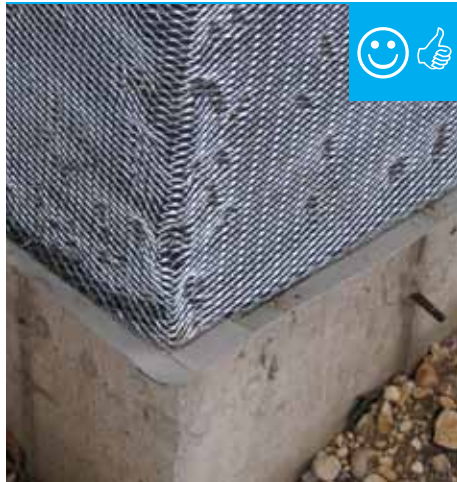
There is a weep screed installed at the bottom of the wall.
