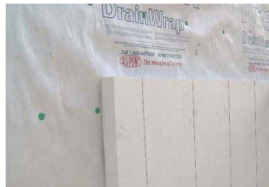
Figure V: DuPont™ Tyvek® DrainWrap® Under Foam Sheathing
