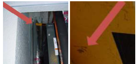
Adding an outdoor air intake vent to the air handler closet delivers fresh air to the conditioned space and improves indoor air quality.
