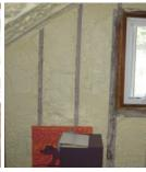
The side attics had a mixture of insulation types, including faced and unfaced fiberglass batt insulation (*left*). These were replaced with closed-cell spray foam on the exterior walls and roof deck to provide a complete and continuous air barrier (*right*), fully aligned with the vapor barrier. This reduced infiltration, mitigating the stack effect, which was pulling warm, moist air up into the attic.
