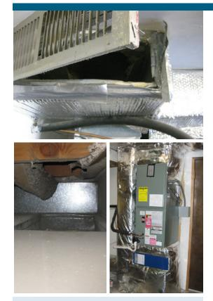
(top) Not only can faulty or poorly placed air returns (such as this one in the garage) allow air infiltration, they can also expose occupants to harmful pollutants.
