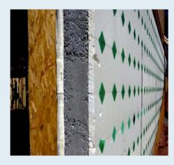
An ICF envelope can be finished with stucco, brick or other materials to produce a desired appearance and add to the aesthetic appeal, as shown below. However, due to the increased wall thickness, the building's footprint is greater than with some other types of framing.
