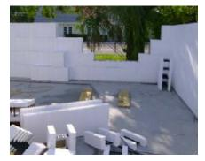
Interlocking pieces are used to create the ICF wall. Concrete is poured onsite into walls of polystyrene foam. Varying thicknesses and materials typically result in R-values between R-20 and R-45. Many times furring strips are used to allow cladding to be easily attached to the exterior.
