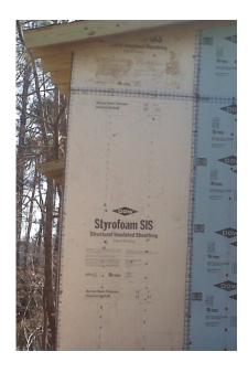
The 2x4 framed wall cavities are filled with R-13 low-density spray foam insulation and then sheathed with moisture-resistant R-3 XPS foam sheathing that is taped to provide a drainage plane and air barrier.
