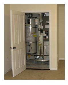
An insulated, conditioned closet within the garage contains the forced-air 92.5% AFUE gas furnace.
