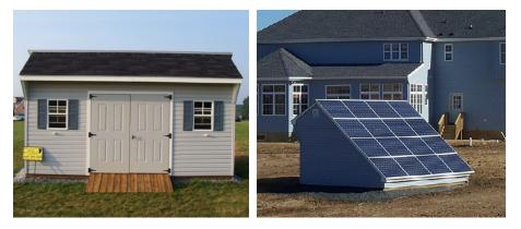
Tindall Homes installed their optional grid-tied solar photovoltaic systems on backyard garden sheds, situated for maximum solar gain. Wiring for the systems runs underground from the shed to the home's basement.
