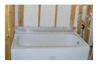
Tommy Williams Homes addresses common thermal bypass issues like heat loss around tubs and showers installed on exterior walls and at attic kneewalls by filling the wall cavities with blown fiberglass and covering them with a rigid air barrier material to prevent heat loss due to air flow.
