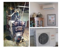
(Left) The original diesel boiler, encapsulated in asbestos, was left in place to eliminate removal and asbestos remediation costs, as well as provide a robust supplemental heating source in extremely cold weather. (Right) The new SEER 16, HSPF 9.4, four-head ductless heat pump system will drastically reduce fuel costs and energy consumption.
