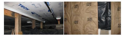
*(left)* In the crawlspace, R-30 fiberglass batts were installed between the 2x10 floor joists. The joists were then covered with 1 inch of expanded polystyrene (EPS) rigid foam board that was taped at the seams to provide a continuous air barrier and flashed at the edges to protect against rodents. The crawlspace floor was covered with a 6-mil visquene vapor barrier.
