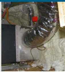
Ceiling drywall was removed along the perimeters of the home to access the attic. Open-cell spray foam was sprayed along the underside of the low-pitch roof to provide an R-21 air sealed, insulated attic space to house the new SEER 16.25 heat pump. (Photo Sources: Calcs-Plus)
