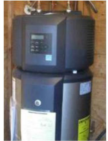
Installing a heat pump water heater in conditioned space can increase energy savings by reducing the load on space conditioning equipment. When there is insufficient room indoors for a heat pump water heater, which requires more clearance than a traditional electric resistance water heater, locating it in the attic or a connected space can also decrease cooling loads by cooling and dehumidifying the attic, the hottest part of the home in summer.
