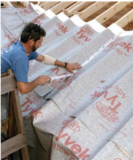
DuPont™ Tyvek® AtticWrap™ is a breathable membrane that helps create a sealed attic system, reducing air leakage and energy loss through the roof.
