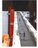
Screed off the concrete until it is even with the block top and then "wet set" anchor bolts into the concrete top.
