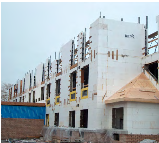
Figure 1 – Best Western hotel constructed using Amvic ICF
