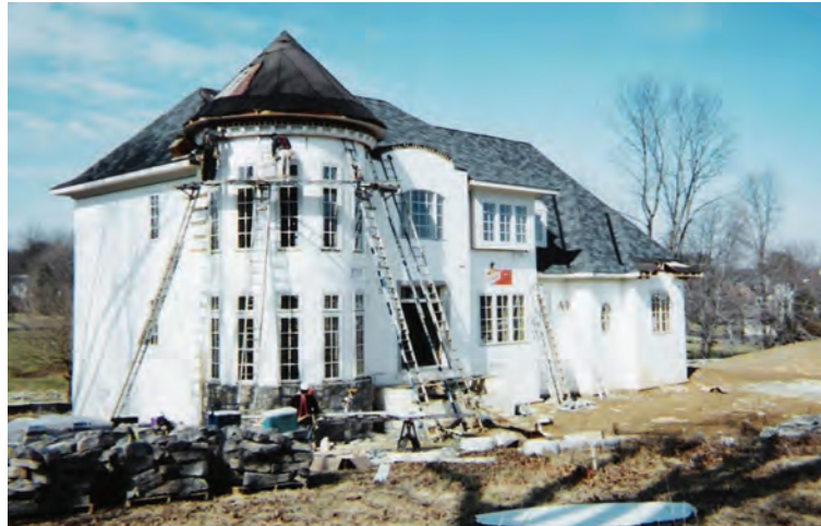
Figure 3 – A custom home being constructed with Amvic ICF
