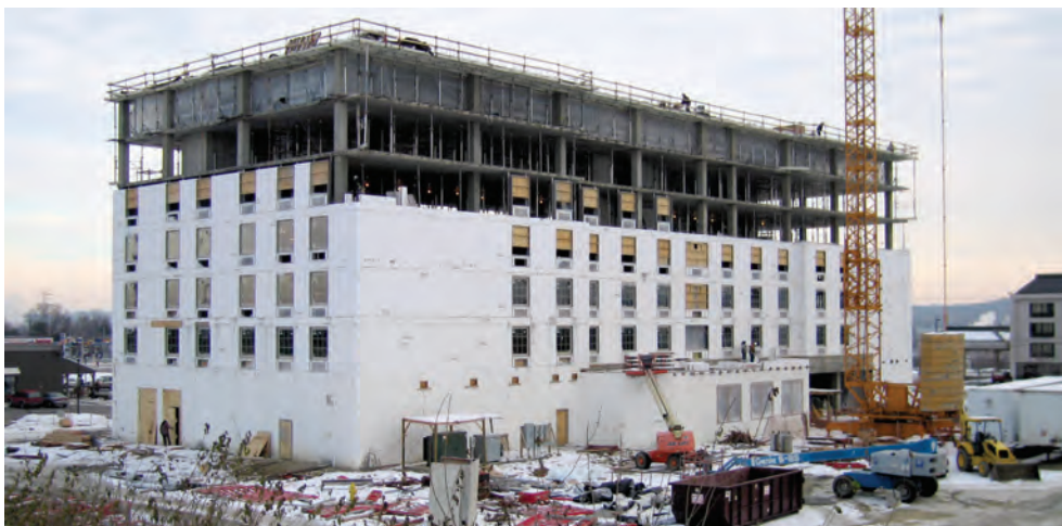
Figure 4 – A multi-storey hotel being constructed with Amvic ICF
