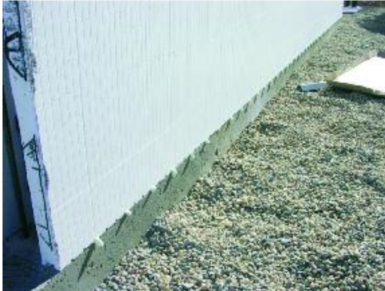
Figure 8.20 – Using foam adhesive to secure the first course of block to the foundation/SOG
