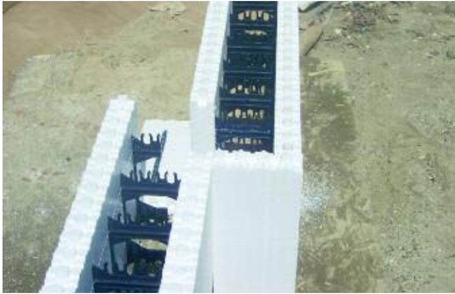
Figure 9.6 – Using cut off pieces to close the open ends and create a corner
