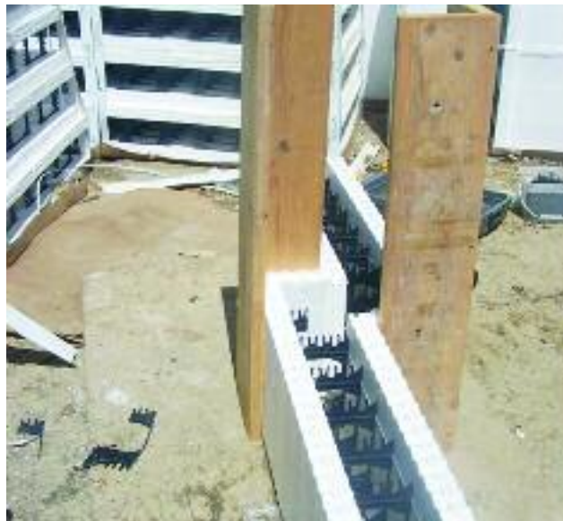
Figure 9.7 – Using 2 x 10 wood forms to support the formed corner
