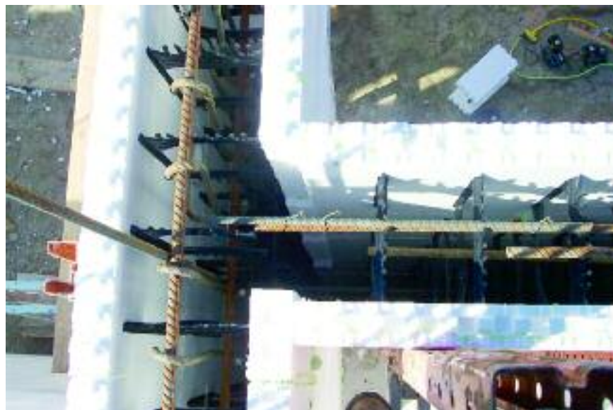
Figure 9.17 – Bracing installed on the exterior side of the T-wall
