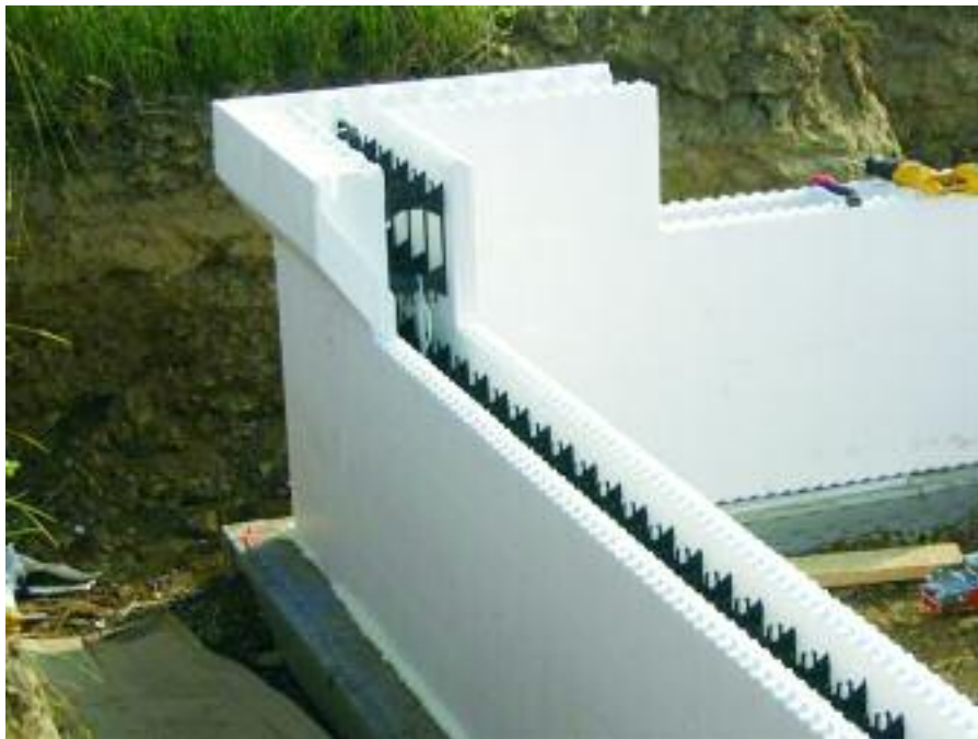
Figure 9.22 – Amvic brick ledge form installed as a single course
