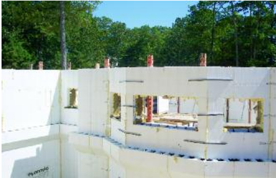
Figure 9.23 – Completed brick ledge installation for exterior brick veneer support
