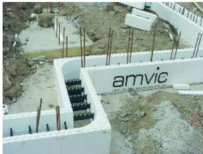
Figure 9.3 – A short corner made of 90° forms with a running bond pattern
