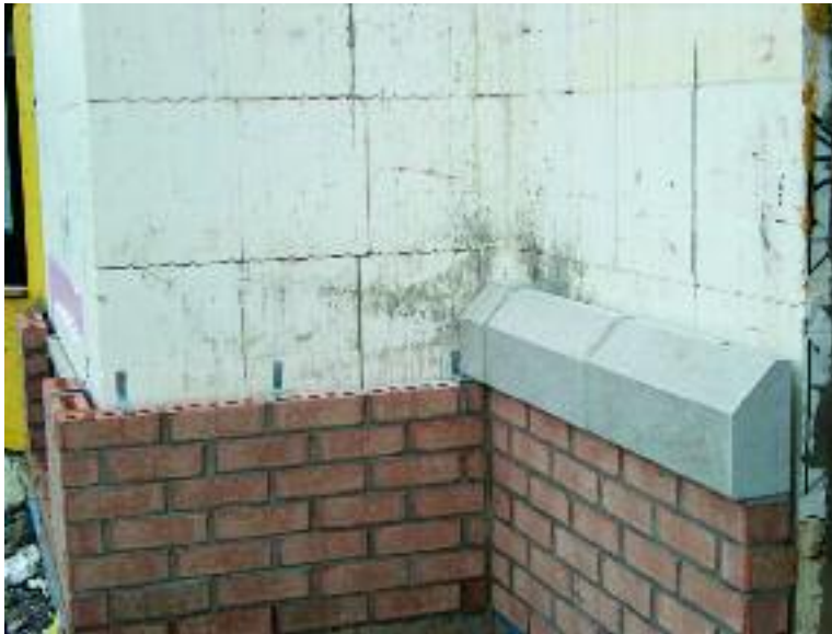
Figure 13.5 – Brick veneer construction on Amvic ICF
