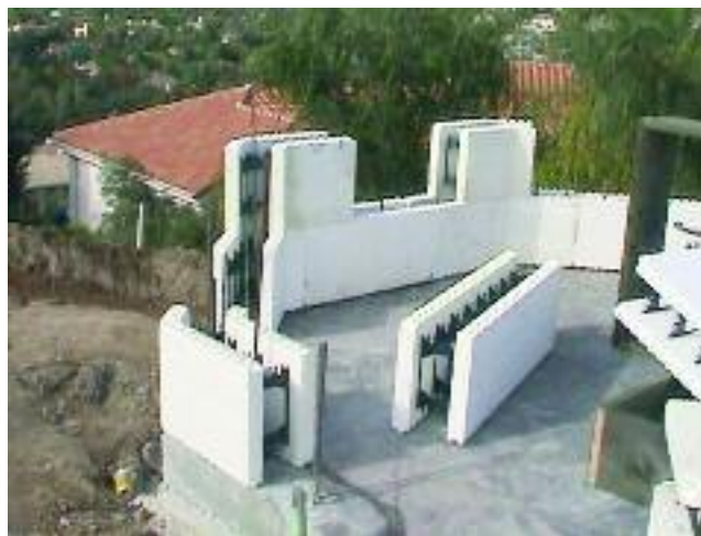
Figure 8.15 – Reversing 45 degree corner blocks for bay window
