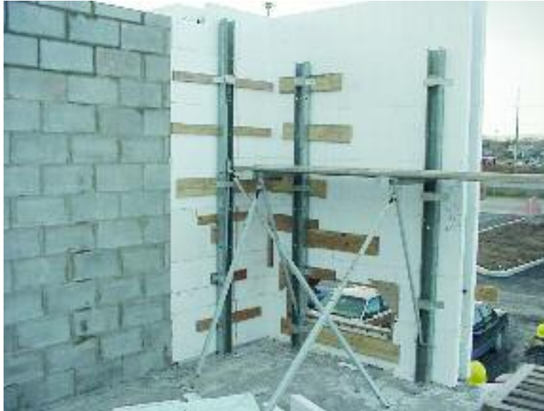
Figure 8.32 – Bracing corners on the inside
