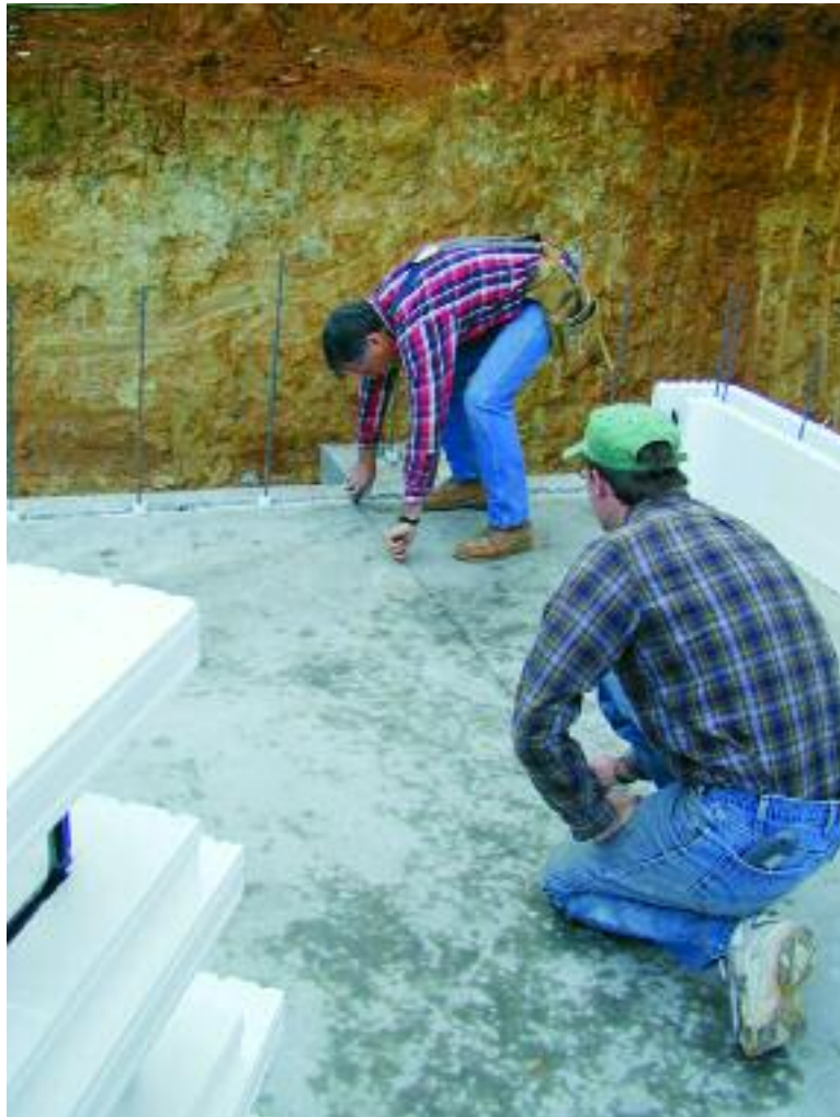
Figure 7.4 – Snap a chalk line to mark your wall Layout
