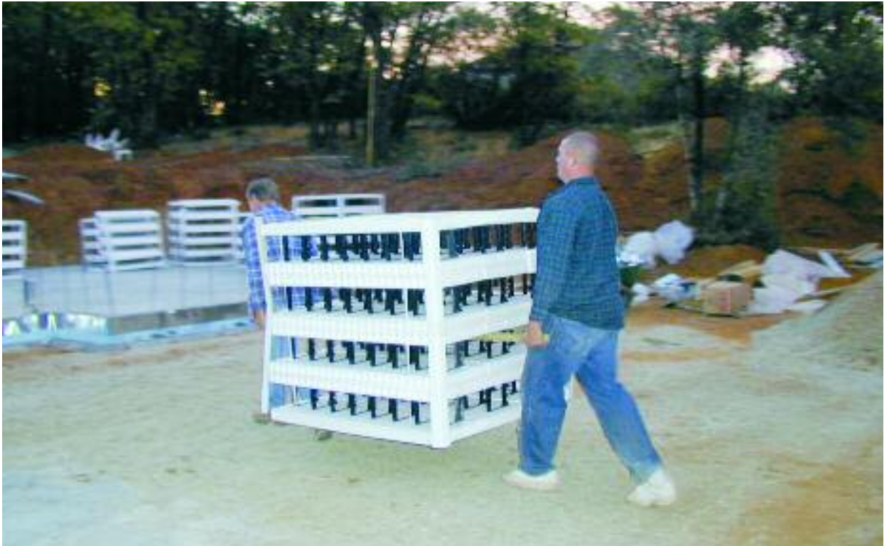
Figure 8.3 – Moving ICF bundles by hand
