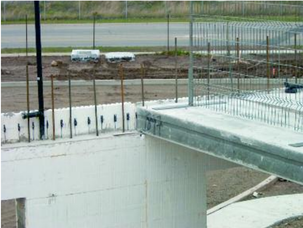
Figure 9.31 – A pre-cast slab panel placed on an ICF wall
