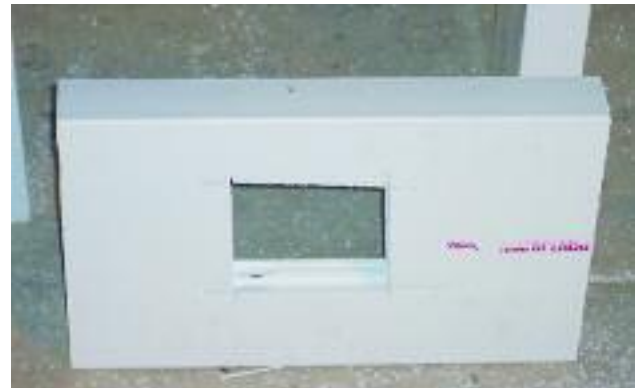
Figure 5.12 – Bottom buck is ready for pouring concrete
