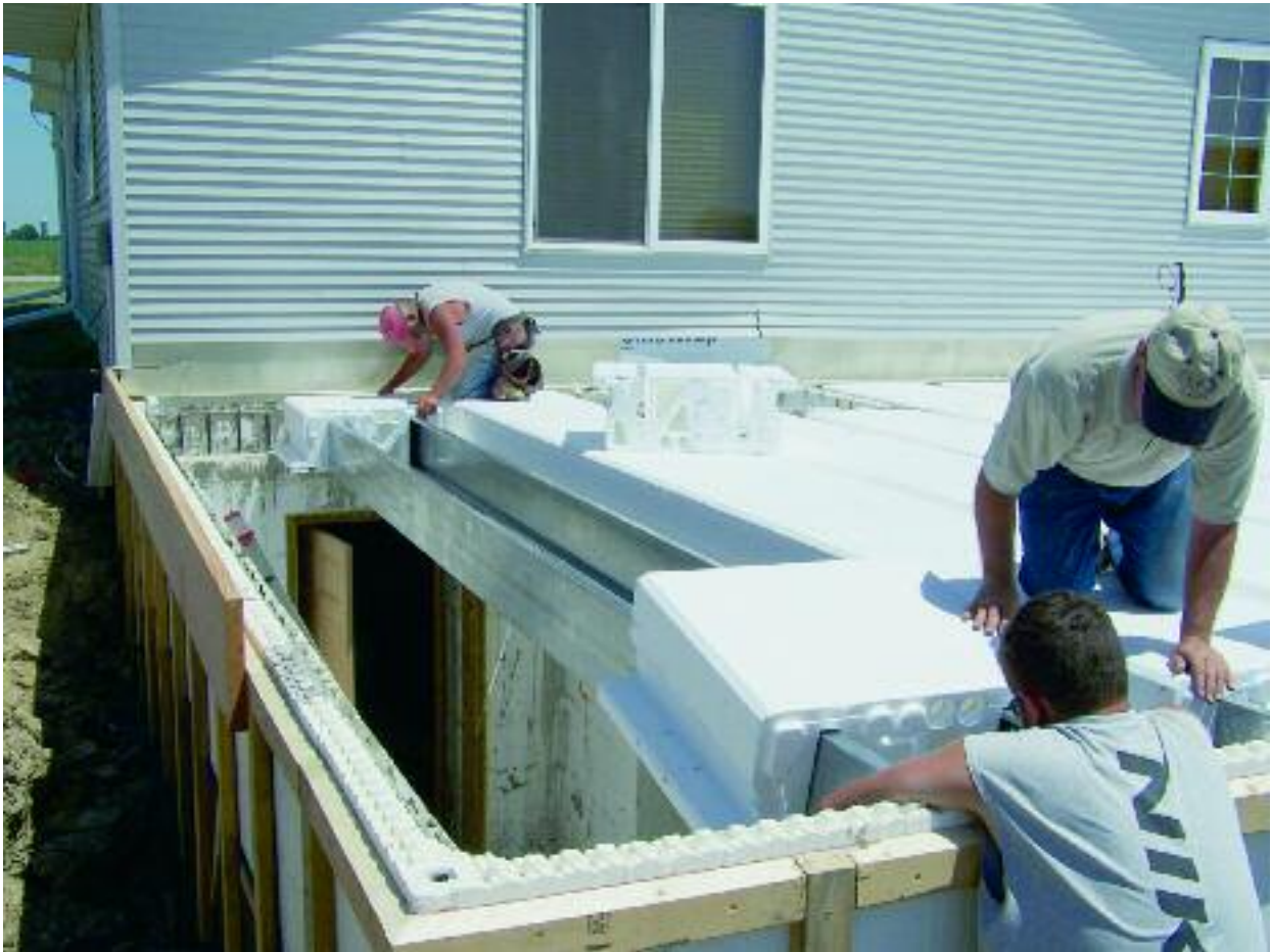
Figure 9.36 – Installing the AmDeck® Floor and Roof System
