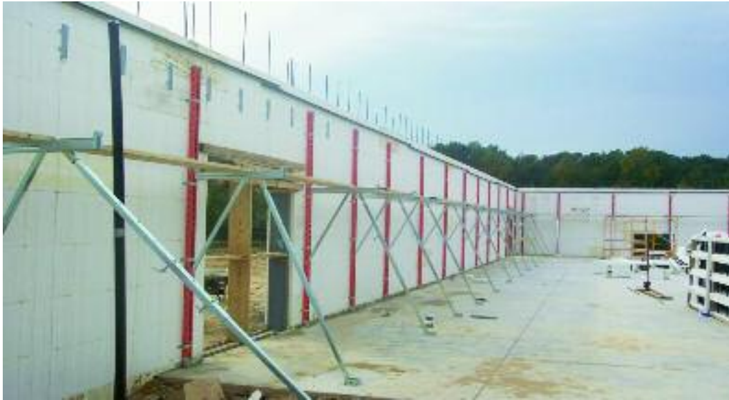
Figure 8.29 – Bracing the inside of the wall
