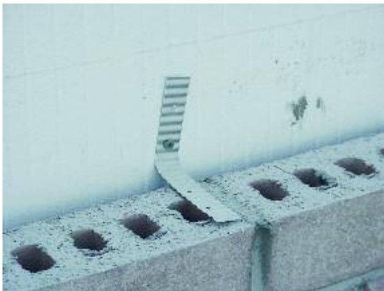
Figure 9.28 – Standard brick ties screwed into the Amvic webs
