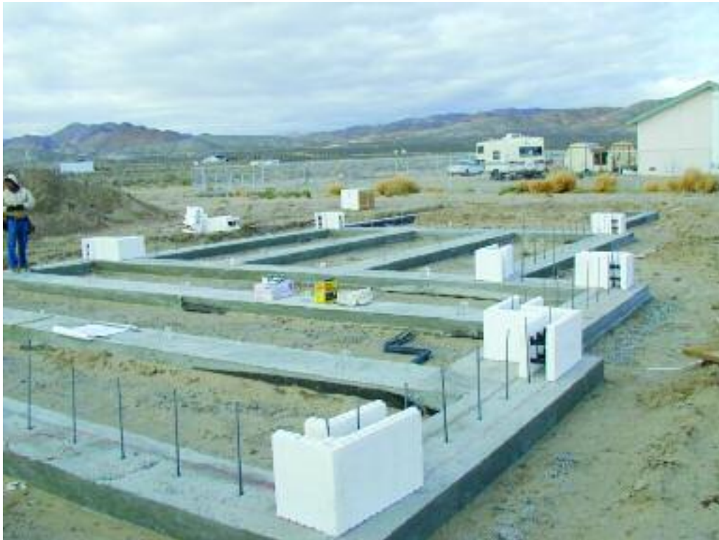
Figure 8.8 – Placing corners first
