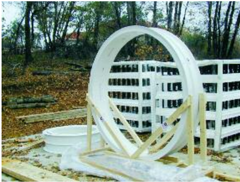
Figure 5.8 – Round openings can be formed easily using vinyl bucks
