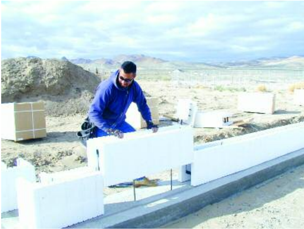
Figure 8.9 – Placing straight blocks
