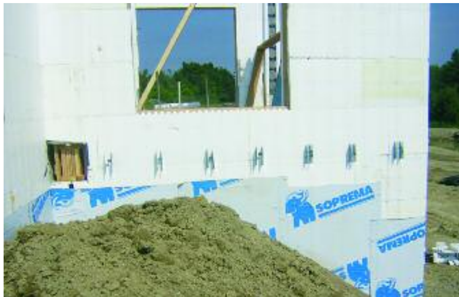
Figure 12.4 – Peel and stick waterproofing membrane installed and ready to be backfilled
