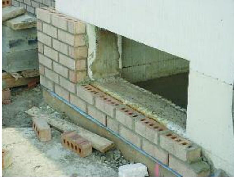
Figure 9.27 – Laying standard brick veneer on the brick ledge support
