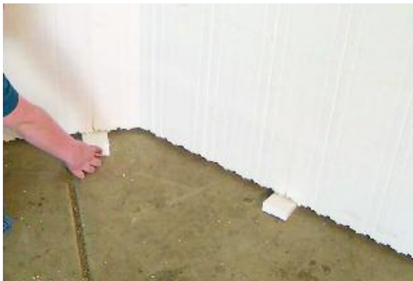
Figure 8.18 – Shimming the first course with foam cuttings
