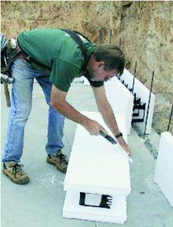
Figure 8.10 – Cutting the final block for a wall section
