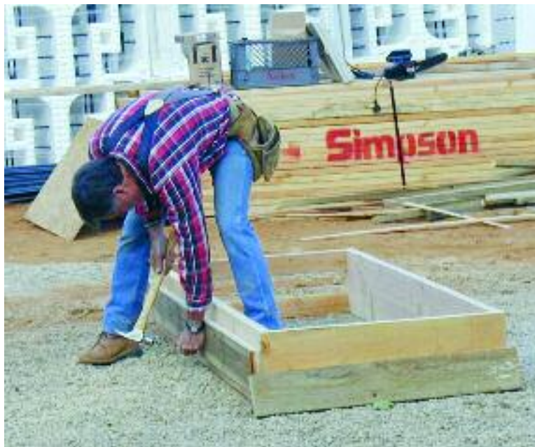
Figure 5.1 – Constructing window/door bucks
