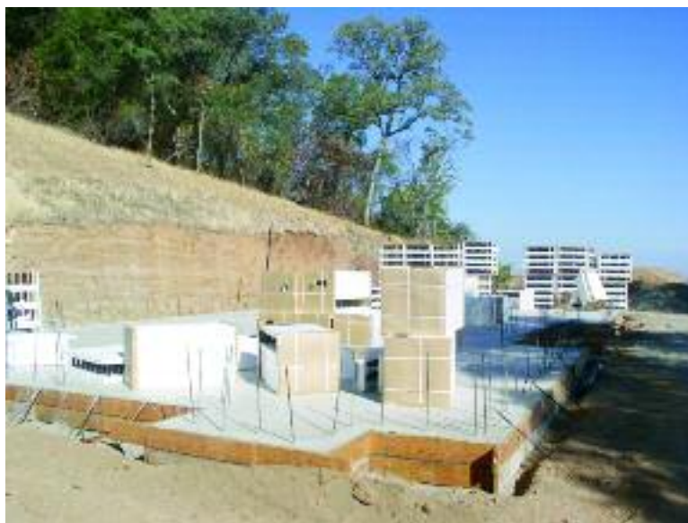
Figure 8.1 – Placing Amvic ICF within the perimeter of the wall layout
