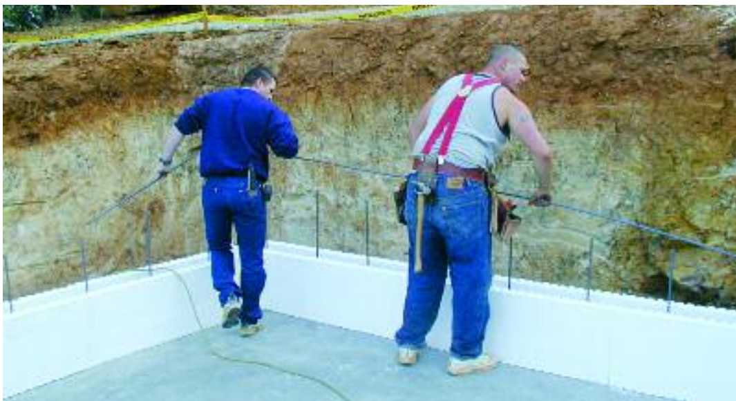
Figure 8.13 – Installing horizontal rebar
