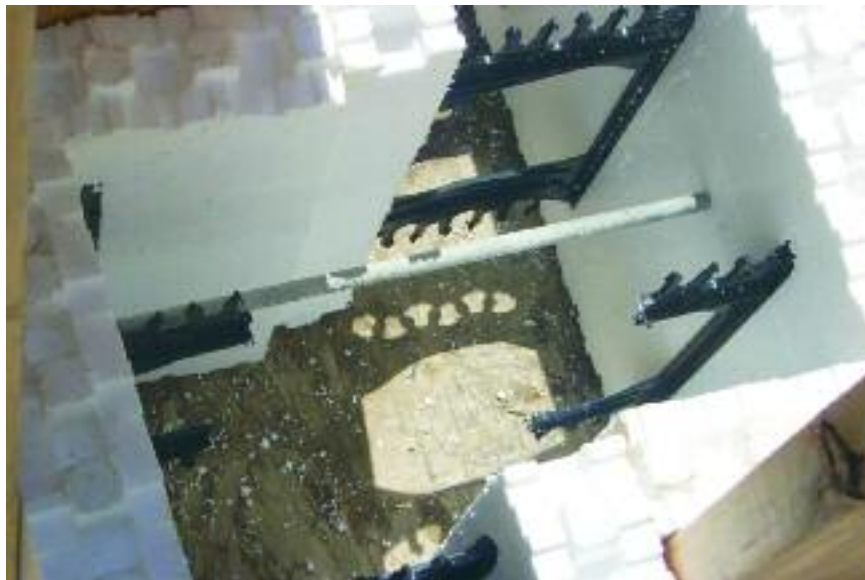
Figure 9.9 – Threaded rod inserted through both wood forms.
