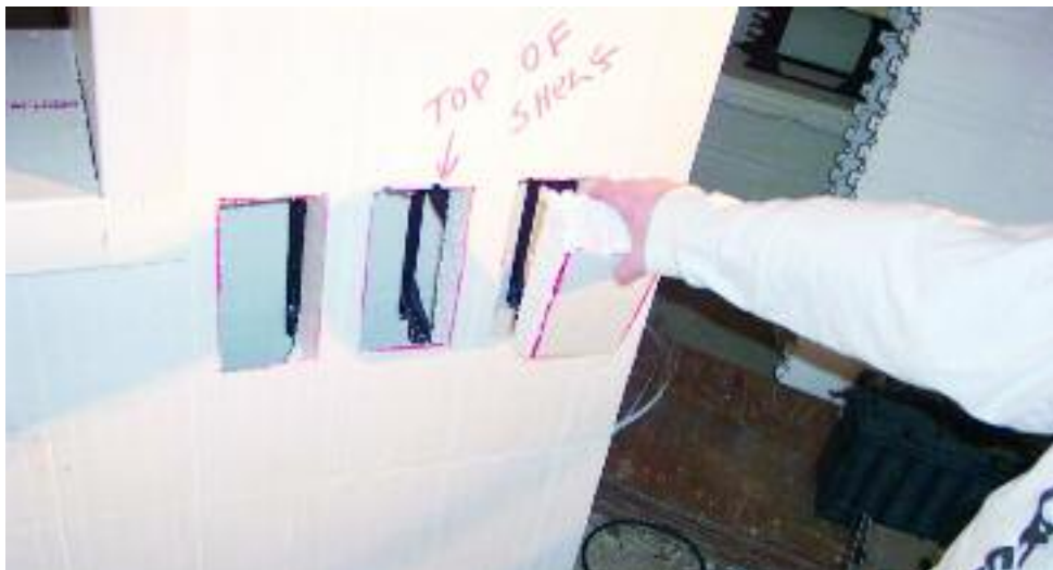
Figure 9.24 – Cutting out EPS between webs
