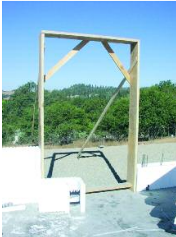
Figure 8.7 – Placing Door Bucks
