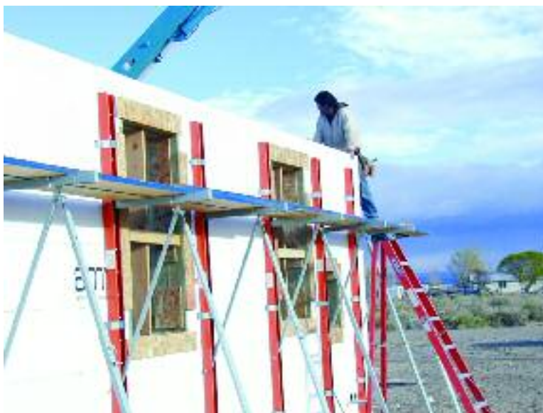
Figure 8.33 – Bracing both sides of wall openings
