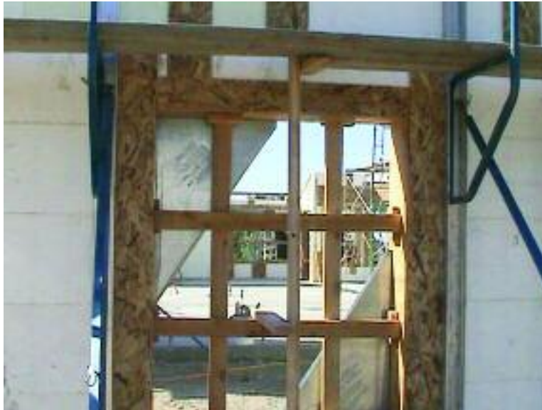
Figure 8.37 – Bracing wall opening vertically and horizontally
