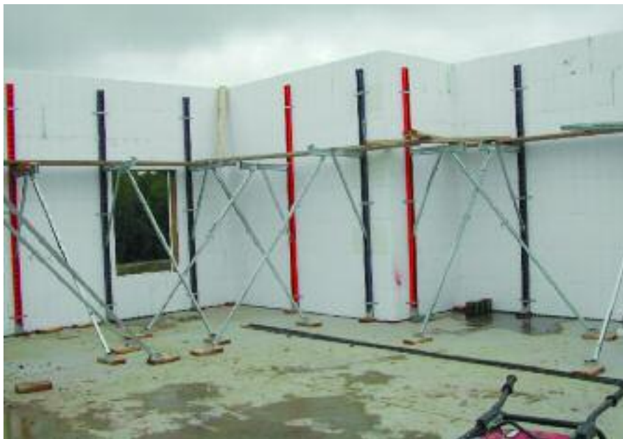
Figure 8.28 – Plumwall bracing & alignment system
