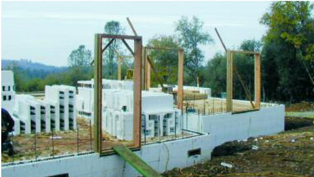
Figure 8.23 – Installing door bucks on the second floor
