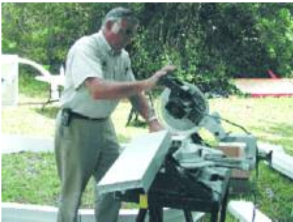
5.10 – Cutting vinyl bucks to required size
