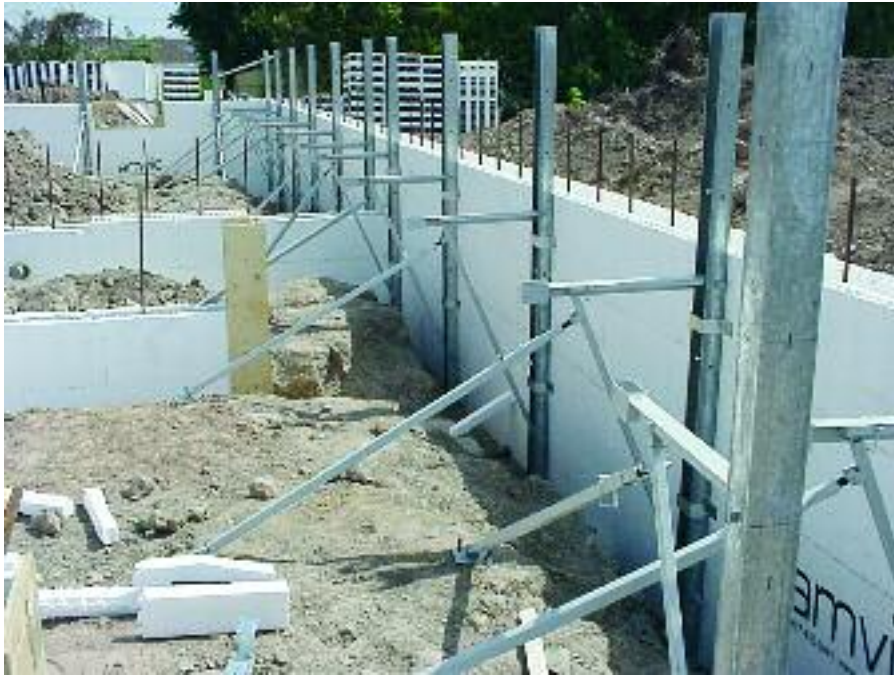
Figure 8.34 – Bracing every 6 feet
