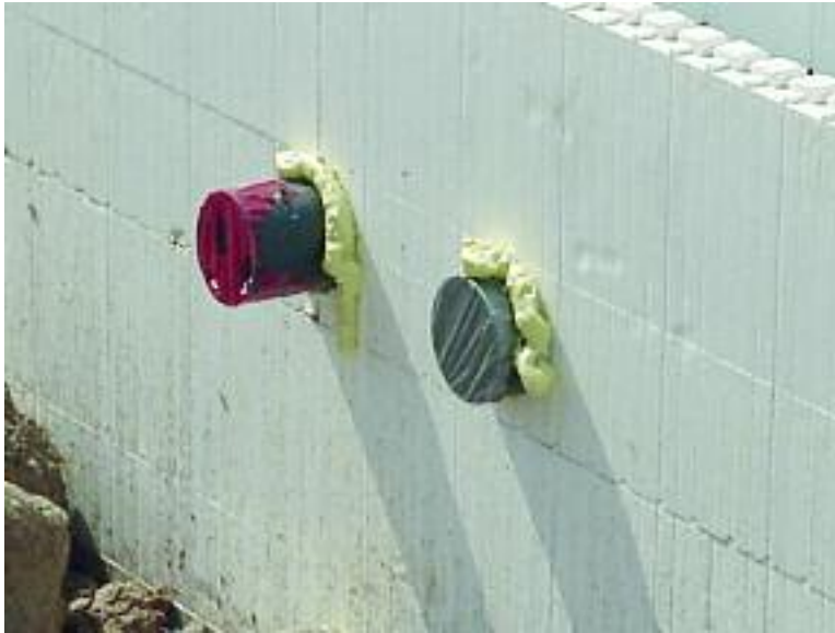
Figure 8.41 – Using PVC pipe for penetration block-outs
