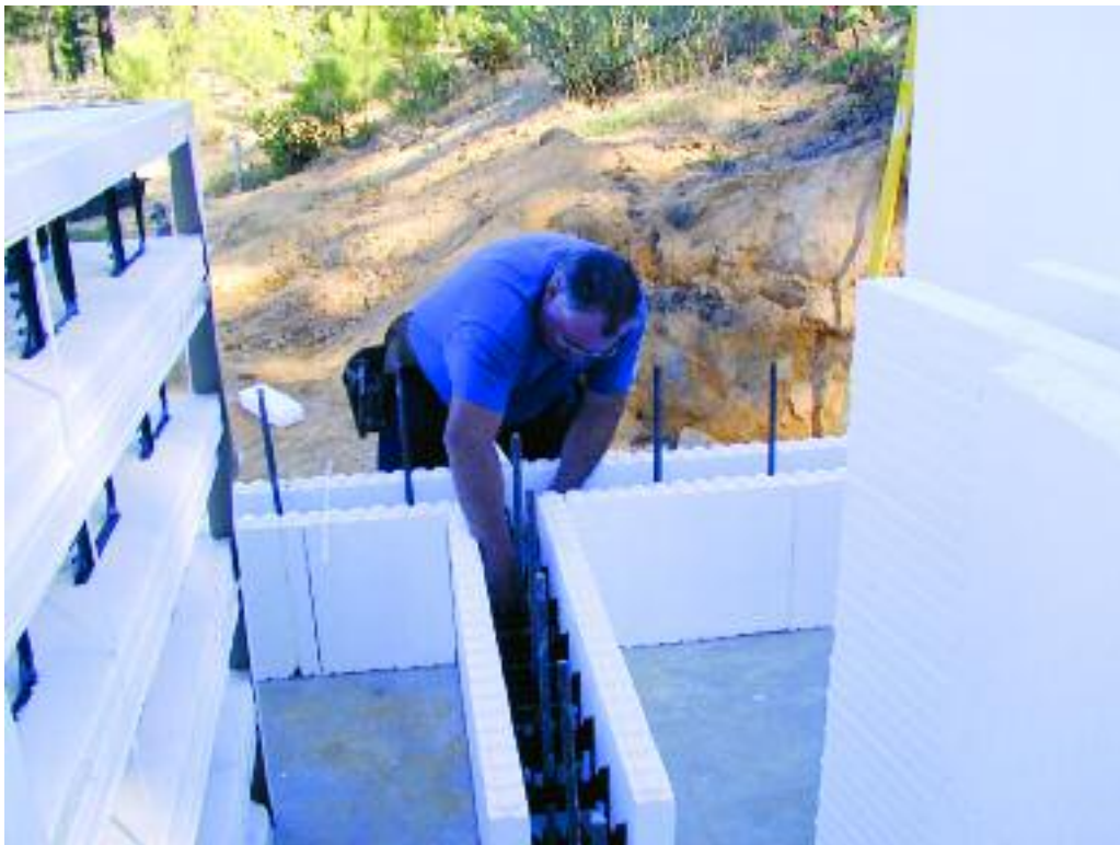
Figure 9.15 – Placing the cut forms together and tying intersecting blocks to form a T-wall. Use metal or plastic wire ties supplied by Amvic
