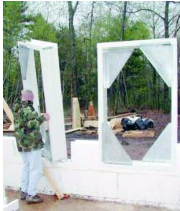
Figure 5.17 – Placing the complete buck in appropriate place. Image courtesy of V-Buck
