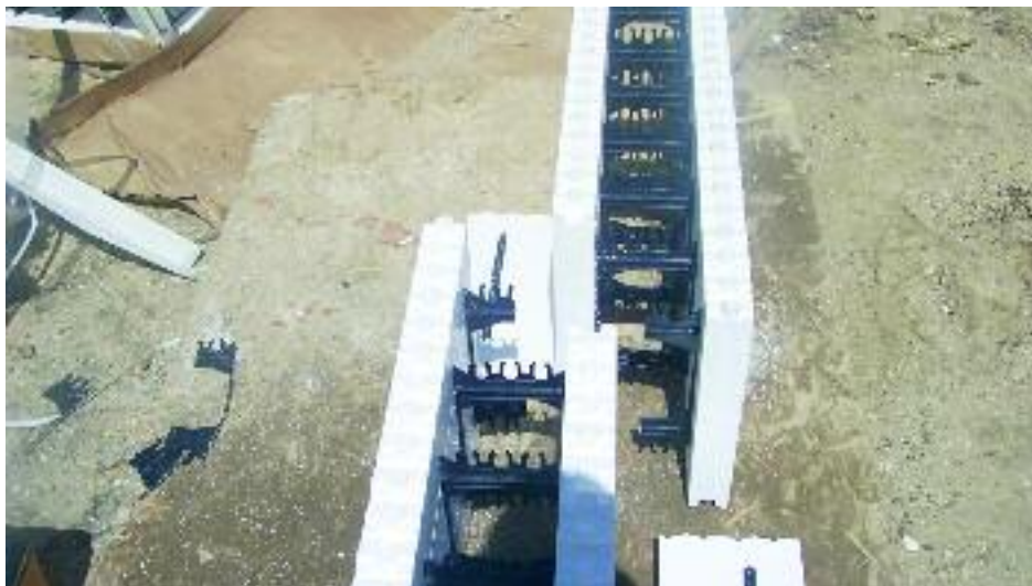
Figure 9.5 – Setting the two cut forms into position
