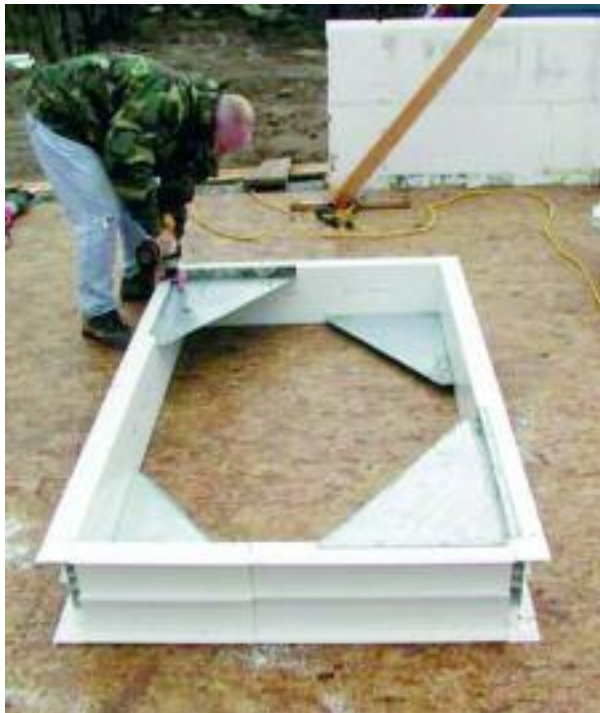
Figure 5.16 – Bracing the bucks with metal corner pans. Image courtesy of V-Buck
