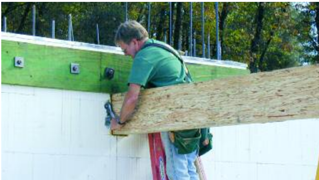
Figure 8.56 – Maneuvering wood beam in place to bear on beam pocket
