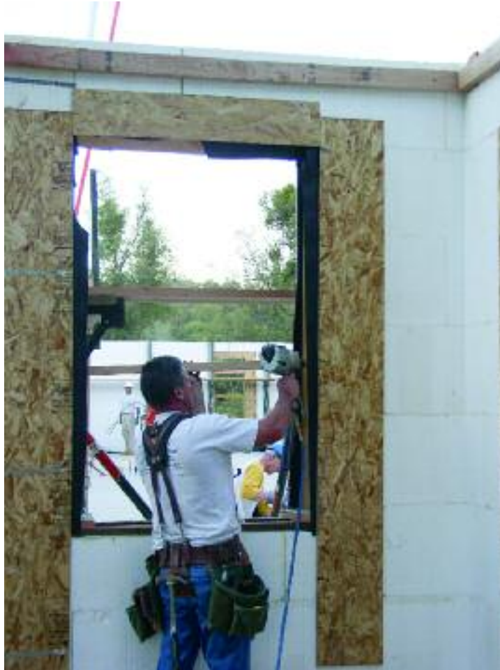
Figure 8.40 – Cleat installation around a door opening using OSB
