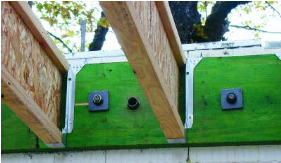
Figure 8.47 – Installing ledger board with proper nuts and washers
