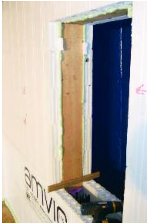
Figure 8.35 – Filling gaps between bucks and forms with foam adhesive
