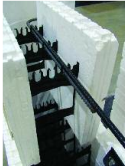
Figure 4.3 – Installing horizontal reinforcing steel and lap splicing
