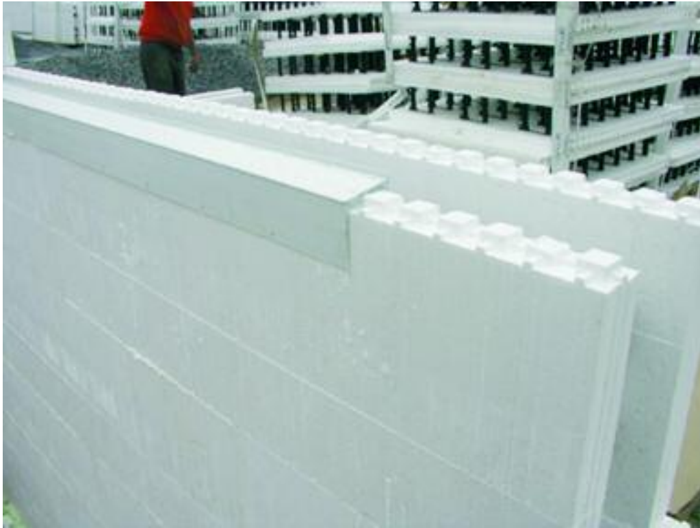
Figure 8.26 – Protecting the Interlock on a top course
