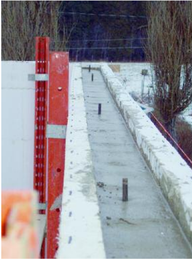
Figure 4.10 – Wet set anchor bolts in top course of upper floor
