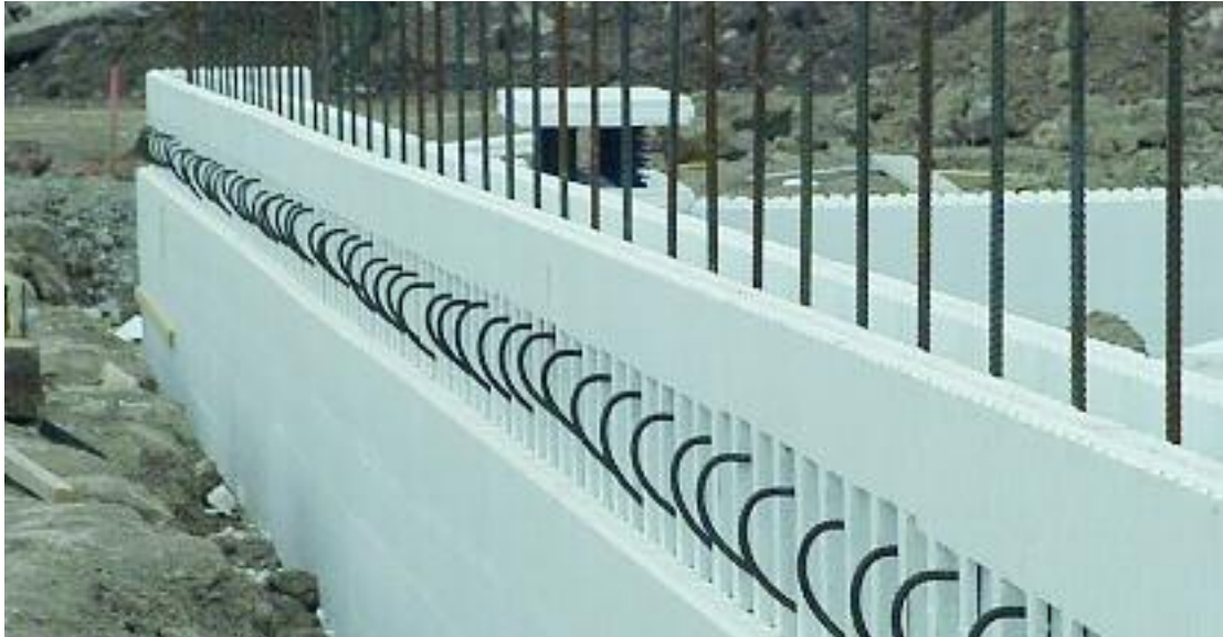
Figure 9.25 – Placing pre-bent brick ledge stirrups
