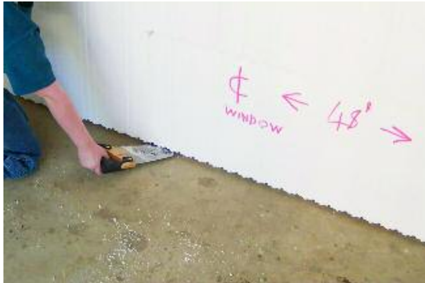
Figure 8.19 – Trimming the first course of block with a hand saw
