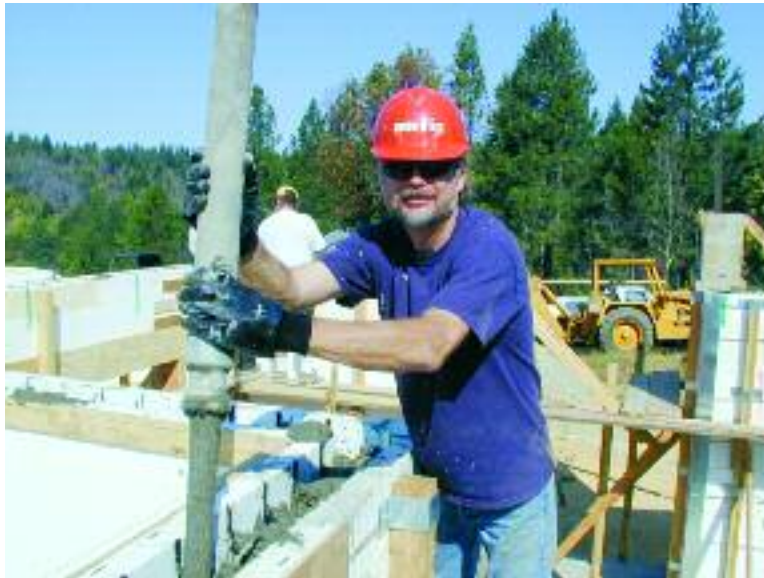
Figure 4.9 – Pouring concrete in lifts of 3-4 ft (0.9-1.2m)
