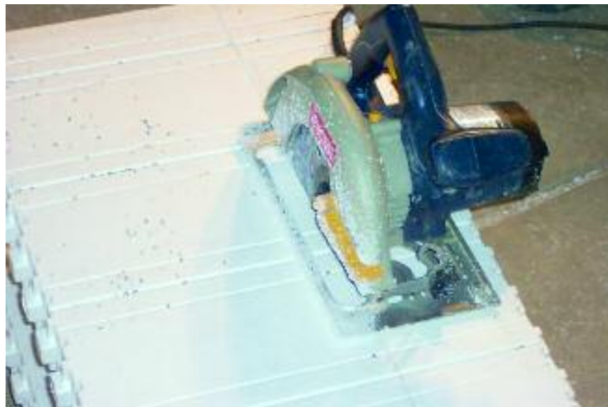
Figure 8.5 – Using a circular saw to horizontally rip cut ICF
