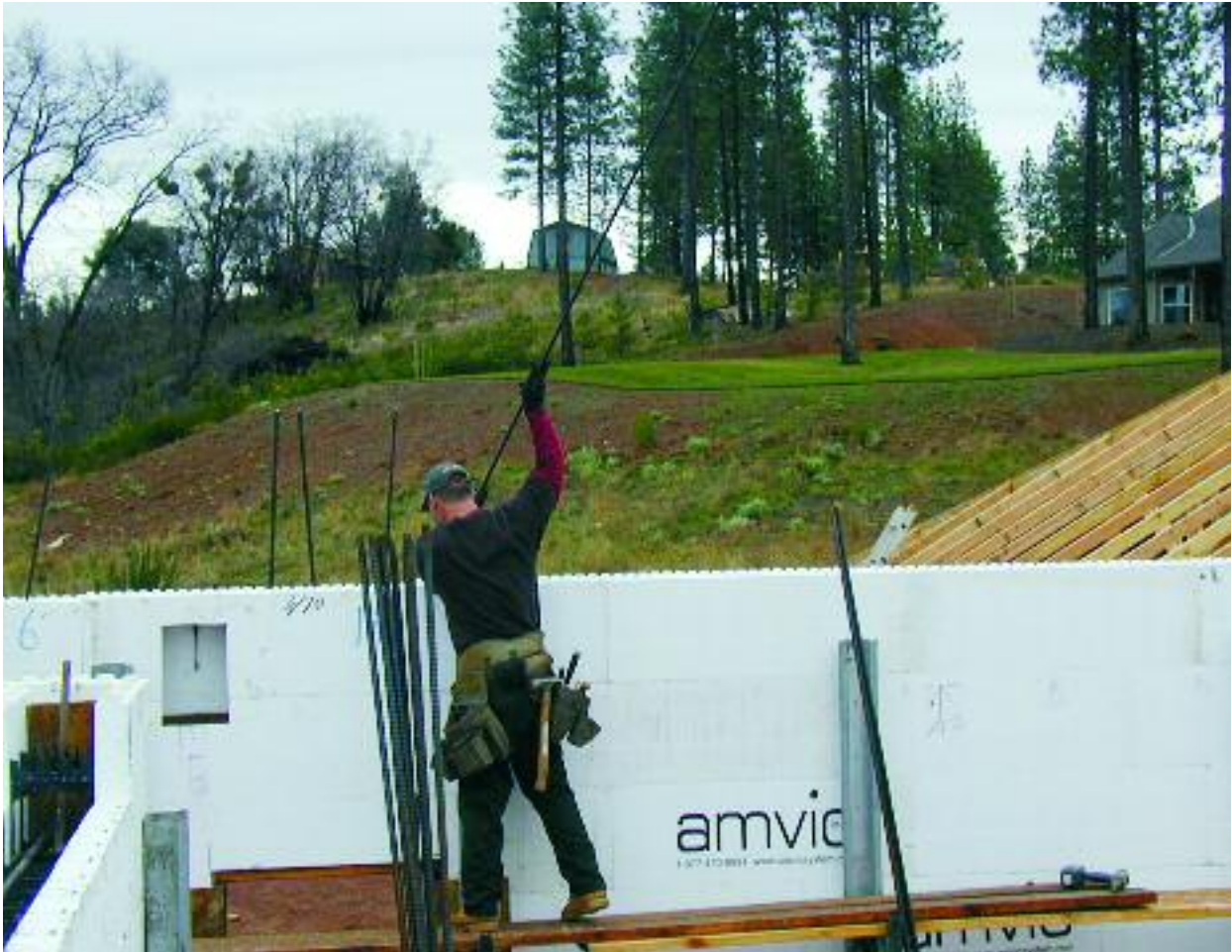
Figure 8.27 – Installing vertical reinforcing steel
