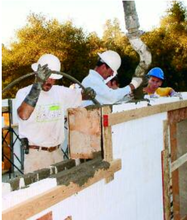
Figure 11.4 – Using internal vibrator to consolidate concrete
