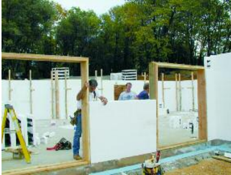
Figure 4.5 – Installing window and door bucks
