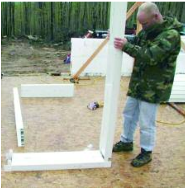
Figure 5.14 – Attaching side pieces to the sill. (Hole for pouring concrete not shown.) Image courtesy of V-Buck
