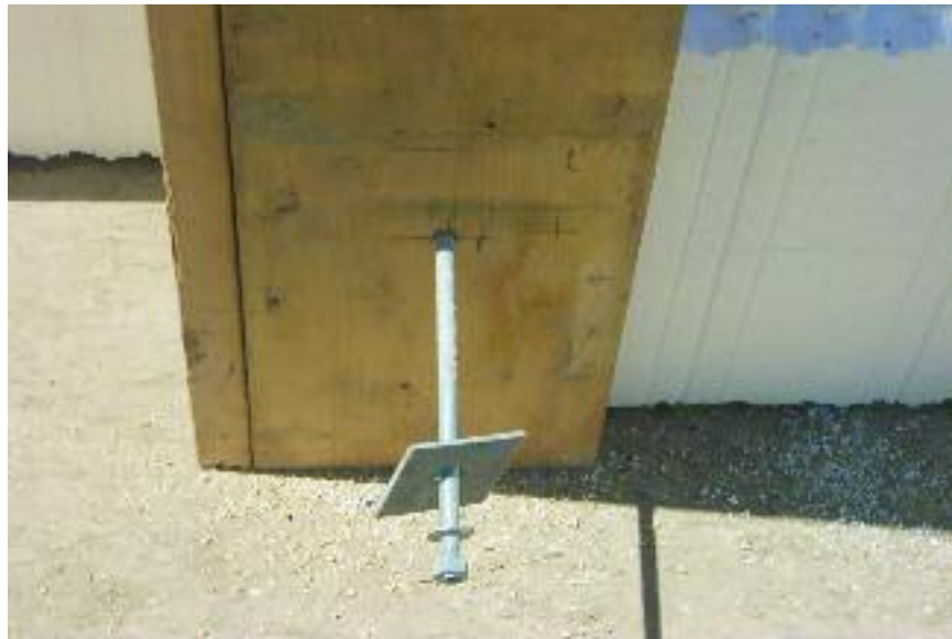
Figure 9.8 – Inserting the threaded rod through the drilled holes
