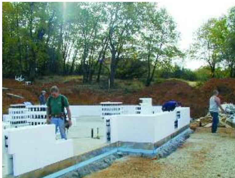
Figure 4.4 – Installing second course of ICF
