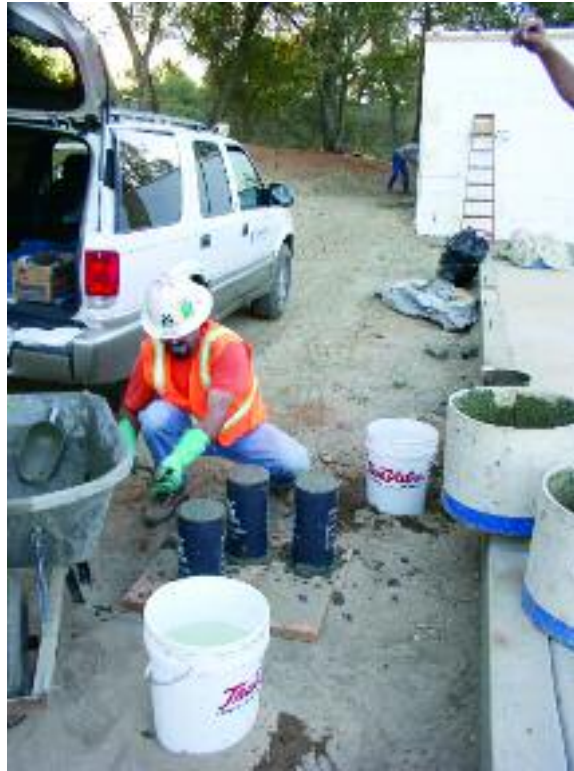
Figure 11.6 – Random sampling of concrete for compressive strength testing at 28 days
