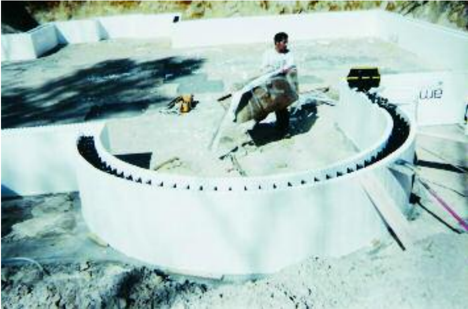
Figure 9.12 – Several courses of Amvic pre-cut radius blocks installed
