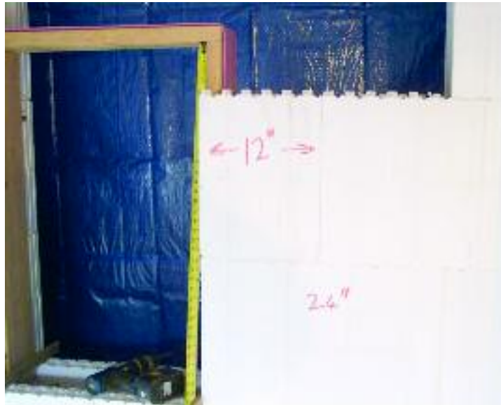
Figure 8.24 – Building courses around window bucks
