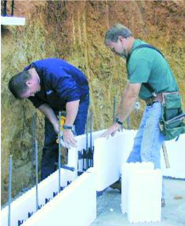
Figure 8.11 – Fitting the cut block in place
