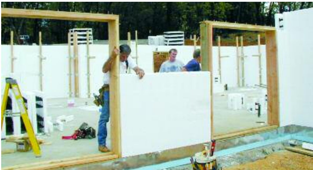
Figure 8.22 – Stacking courses around door bucks
