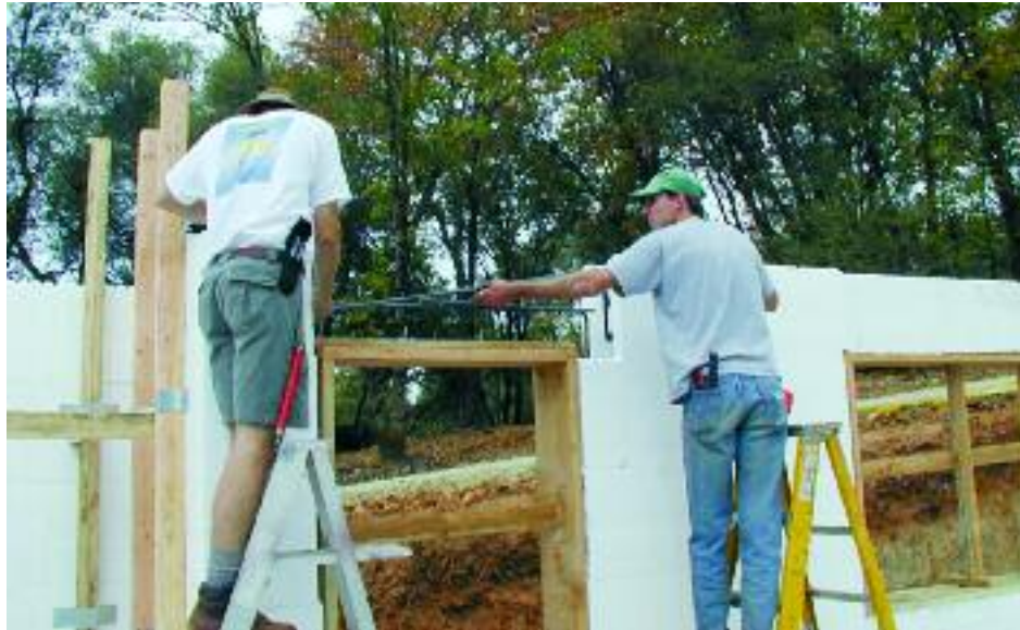
Figure 8.25 – Installing reinforcing steel bars for wall opening header or lintel
