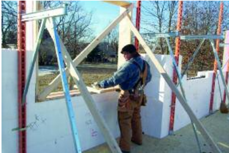
Figure 4.7 – Installing alignment and bracing system around the perimeter of the wall
