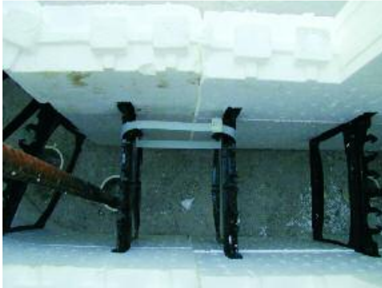
Figure 8.12 – Using zip ties to tie the first course blocks together
