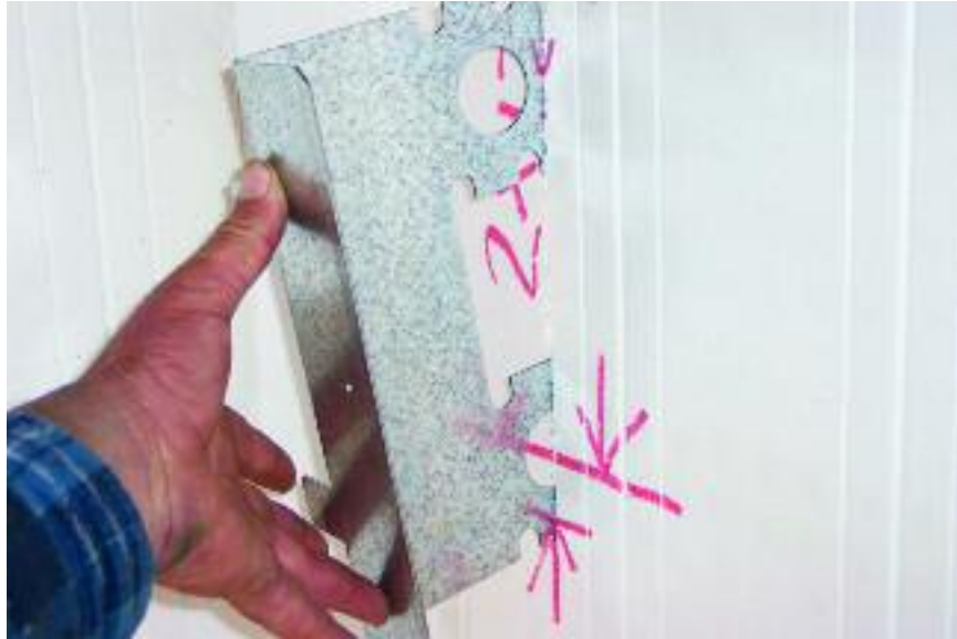
Figure 8.50 – Inserting the ICFLC long blade through the EPS and into the concrete
