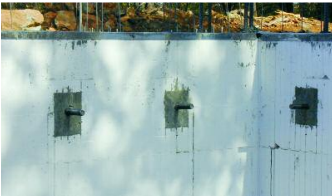
Figure 8.46 – Allowing the concrete to cure for at least 3 days before removing the OSB square pieces
