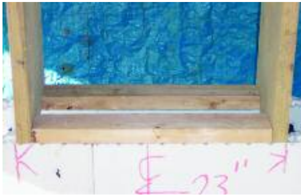
Figure 5.4 – Typical window buck bottom construction
