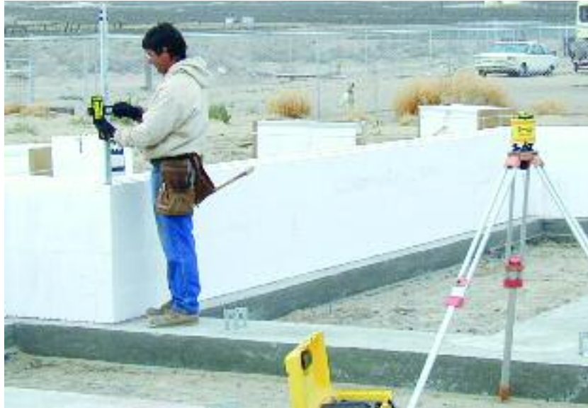
Figure 8.17 – Checking for level after second course placement
