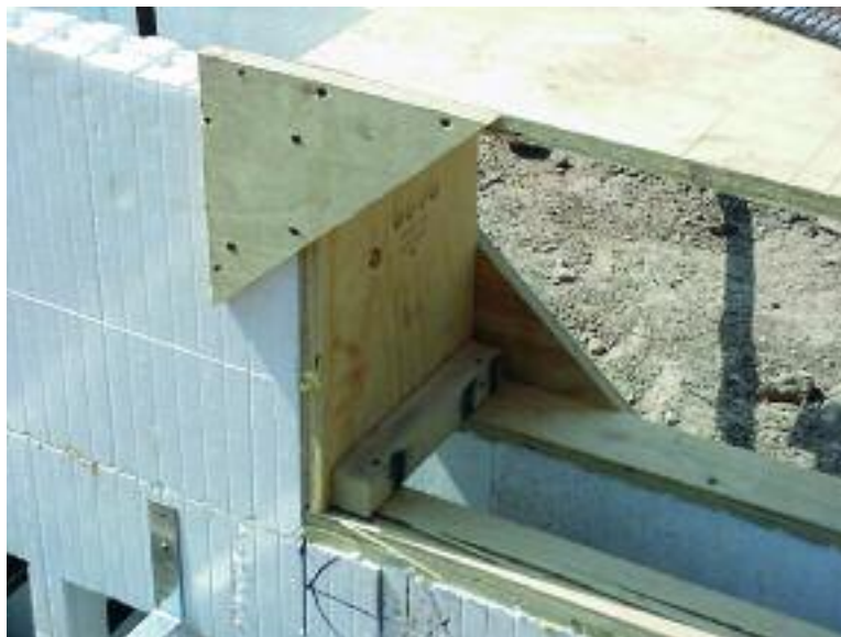
Figure 8.36 – Installing cleats around wall openings
