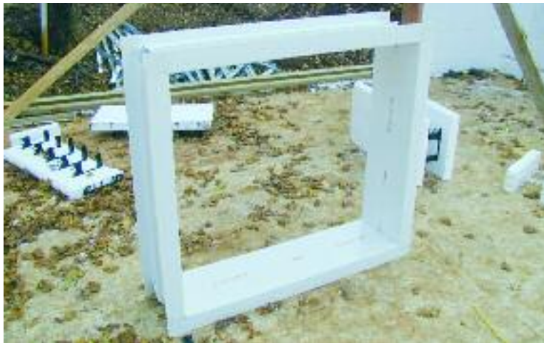
Figure 5.7 – Typical vinyl window buck
