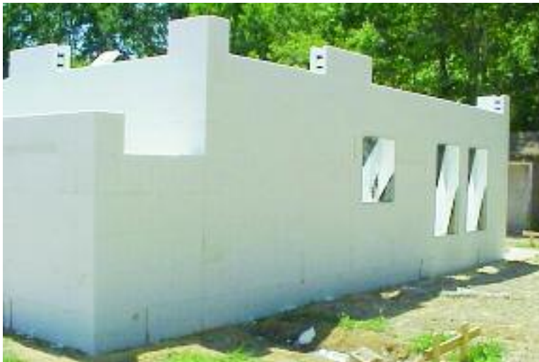
Figure 4.6 – Continuing installing block courses
