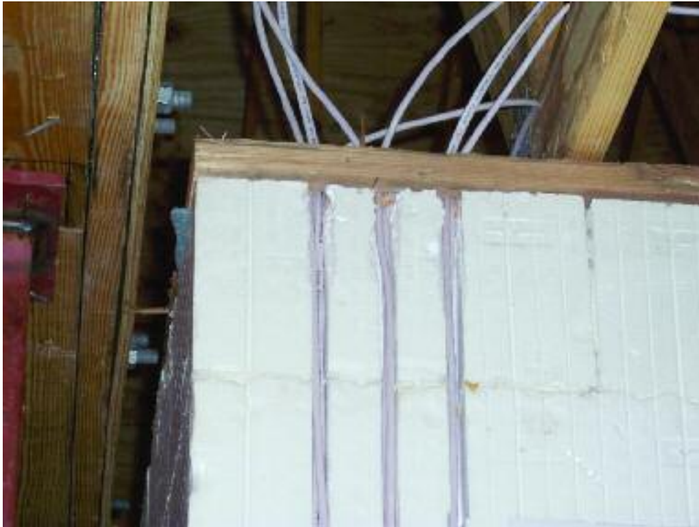
Figure E1.3 – Embedding Romex into the EPS panels
