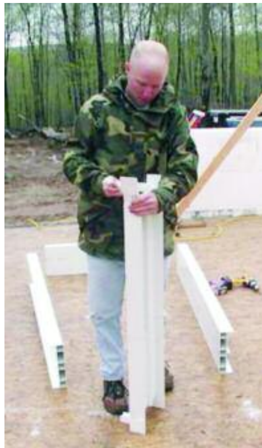
Figure 5.13 – Inserting Connectors. Image courtesy of V-Buck
