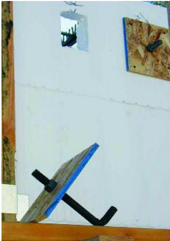
Figure 8.42 – Cutting square OSB boards for anchor bolt installation
