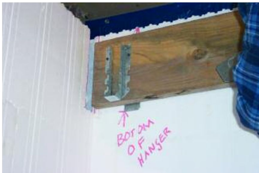
Figure 8.51 – Securing the ledger board in place temporarily
