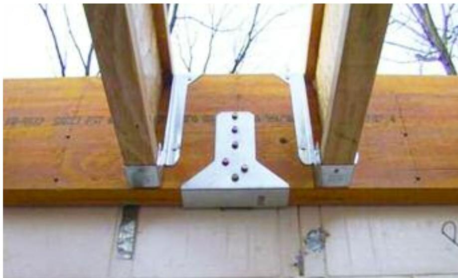
Figure 8.53 – Attaching floor joists to the ledger board with the Simpson Strong-Tie™
