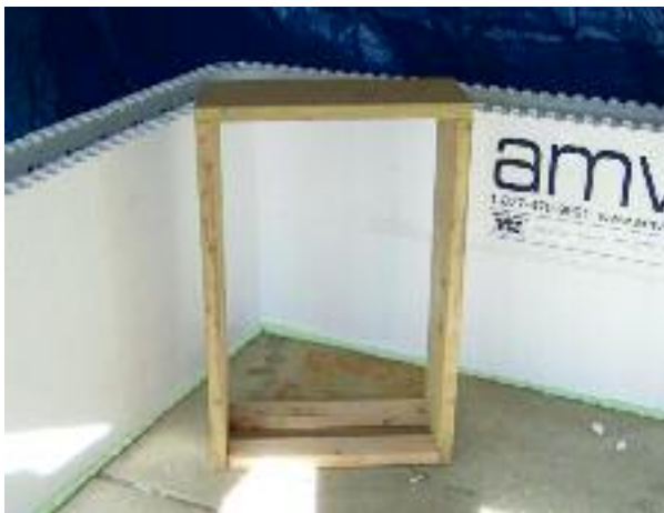
Figure 5.2 – Typical buck made of pressure treated lumber
