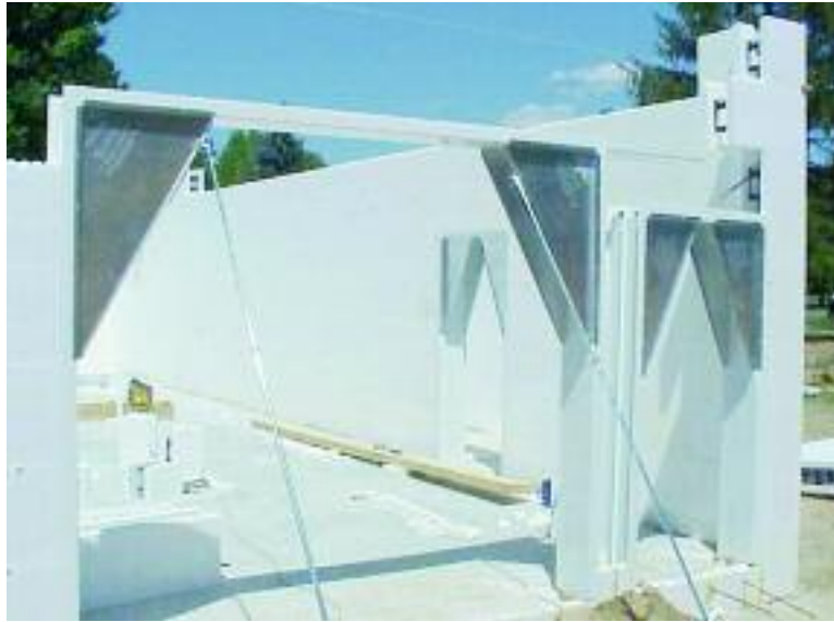
Figure 5.9 – Vinyl bucks come with accessories including bracing pans and connectors
