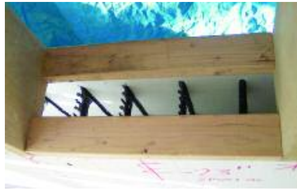
Figure 5.5 – Opening at bottom of window buck for pouring concrete
