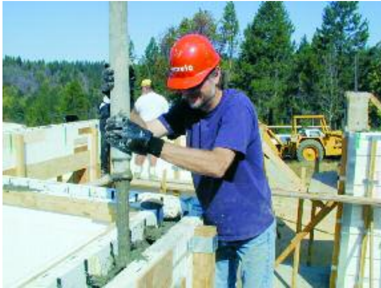
Figure 11.2 – Pouring concrete for 90° Corner
