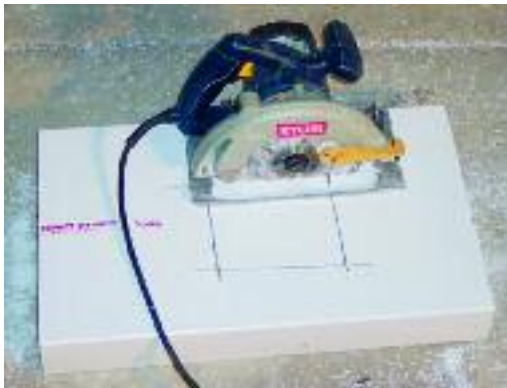
Figure 5.11 – Cutting a hole in bottom buck
