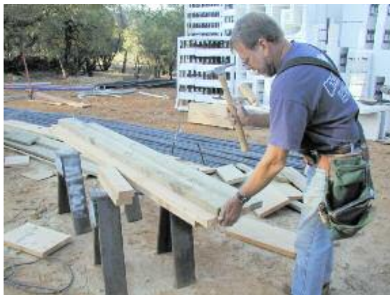
Figure 5.6 – Installing nails into the bucks for attachment to concrete
