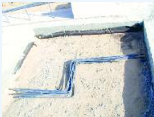
Figure 8.2 – Pre-cut & bent reinforcing steel will increase efficiency
