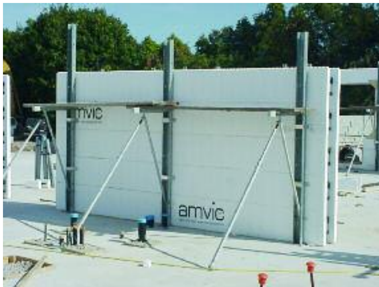
Figure 8.30 –Platform and scaffold planks
