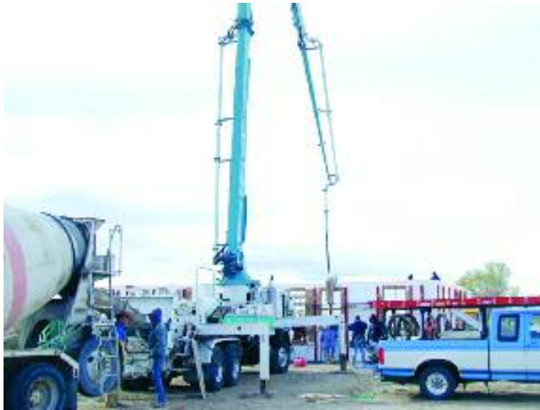
Figure 11.1 – Using boom pump to pour concrete in Amvic ICF
