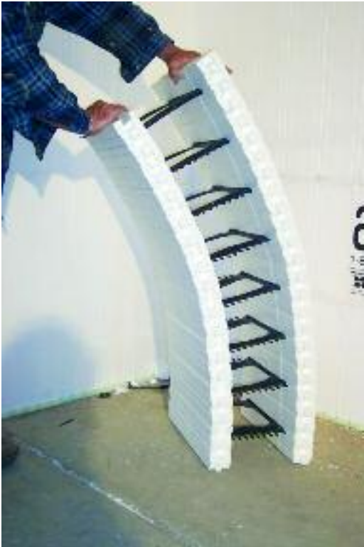
Figure 9.11 – Bending and securing the radius form into place
