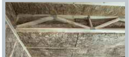
Inner-Safe Concealed Space Batt installed in Open Web interstitial space.
