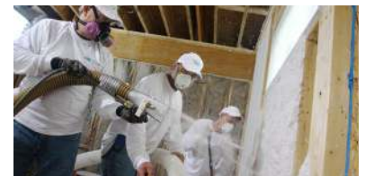
Vacuuming simultaneously with spraying will help to maintain proper moisture density.
