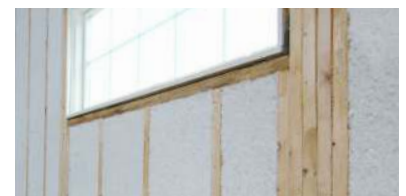
Final cavity should present a clean, well-filled appearance.
