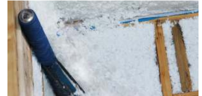
At top of cavity, reverse scrubber direction to push fiber upwards.
