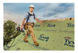
**INDUSTRY-LEADING WALKABILITY** The unique embossed pattern allows for better traction and grip while walking on the roof.
