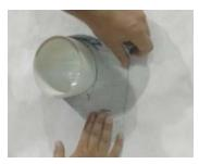
8. Fan out the remaining DuPont<sup>™</sup> FlexWrap<sup>™</sup> EZ onto the WRB around the circumference of the pipe. Use firm hand pressure on both pipe and WRB surfaces for a good bond and a secure seal. If any wrinkles or creases form during application, ensure they are smoothed out and adhered with firm hand pressure.
