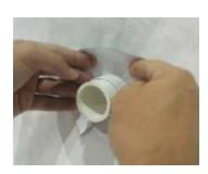
**12.** Use firm hand pressure on both pipe and WRB surfaces for a good bond and secure seal. Remove any wrinkles or creases by using firm hand pressure to ensure a fully adhered and smooth surface.
