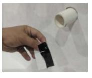
4. While still folded, center DuPont<sup>™</sup> FlexWrap<sup>™</sup> EZ under the pipe and use the remaining release paper edge to position DuPont<sup>™</sup> FlexWrap<sup>™</sup> EZ tight against the WRB. Adhere the exposed butyl to the underside of the pipe.
