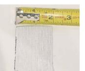
Fold the piece of DuPont<sup>™</sup> FlexWrap<sup>™</sup> EZ to break perforations in release paper to create a 90 degree angle.
