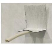
Extend both sides of DuPont<sup>™</sup> FlexWrap<sup>™</sup> EZ below the wire and adhere each corner and outside edge to WRB as shown.
