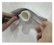
Extend the length of DuPont<sup>™</sup> FlexWrap<sup>™</sup> EZ and gently remove remaining release paper to avoid stretching the product.
