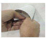
8. Fold the second piece of DuPont<sup>™</sup> FlexWrap<sup>™</sup> EZ to break perforations in release paper and create a sharp crease. Remove narrow (~1") width of release paper. While still folded, center DuPont<sup>™</sup> FlexWrap<sup>™</sup> EZ above the pipe and use the remaining release paper to position tight against the WRB. Adhere the exposed butyl to the top, and down each side of the pipe to the 3 and 9 o'clock positions.
