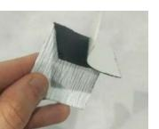
Position DuPont<sup>™</sup> FlexWrap<sup>™</sup> EZ above the wire so the exposed butyl is centered on top of the wire, and the side with remaining release paper is against the WRB.
