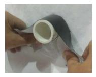
Fan out the remaining unadhered DuPont<sup>™</sup> FlexWrap<sup>™</sup> EZ onto the WRB above and down each side of the pipe.
