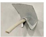
6. Pinch together the exposed butyl of DuPont<sup>™</sup> FlexWrap<sup>™</sup> EZ below wire to create a flap and complete a full perimeter seal around wire. Use firm hand pressure to remove any pinholes at the crease below the wire where the butyl is adhered together.
