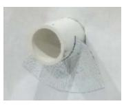
Cut a second piece of DuPont<sup>™</sup> FlexWrap<sup>™</sup> EZ the length of the pipe circumference.
