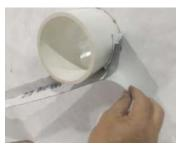
7. Unfold and fan out DuPont<sup>™</sup> FlexWrap<sup>™</sup> EZ applied at the 3 o'clock position to the WRB. Adhere the remaining exposed butyl of DuPont<sup>™</sup> FlexWrap<sup>™</sup> EZ to lap over the layer below and then onto the WRB.
