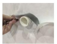
Position the unadhered butyl of the narrow section below to overlap the edges of DuPont<sup>™</sup> FlexWrap<sup>™</sup> EZ installed first by a minimum of 1". Use thumbs to adhere. Do not stretch DuPont<sup>™</sup> FlexWrap<sup>™</sup> EZ.
