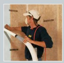
Jet Stream® **ULTRA** is an excellent product for Blow-in-Blanket applications. It will dense-pack in wall cavities with no settling.
